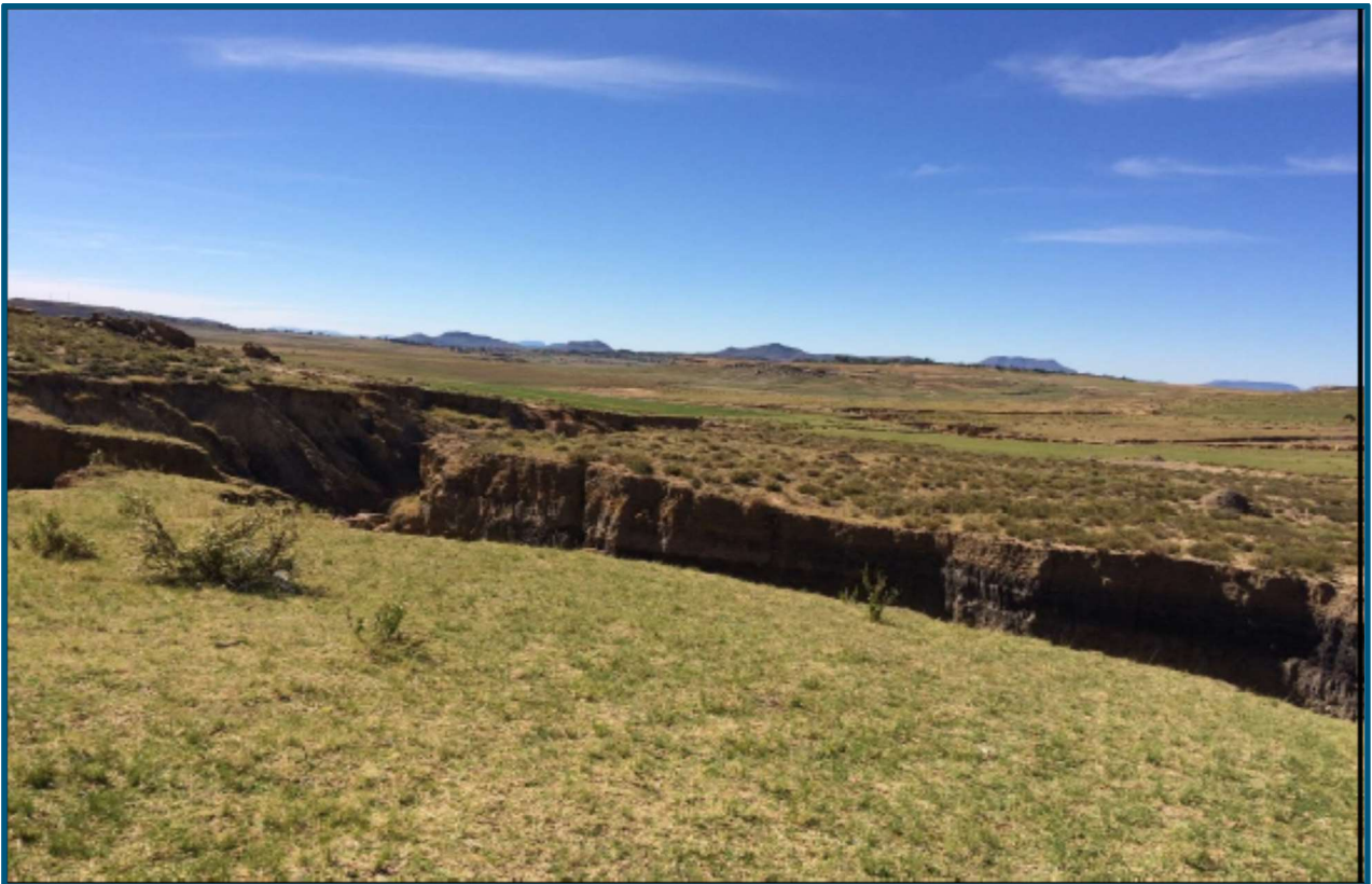
Figure 24: Eroded Upstream Section of the Main River
