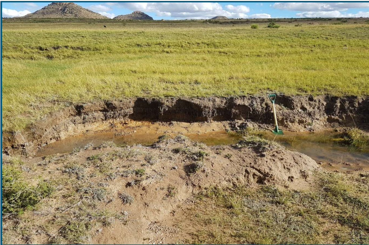
Figure 84: Example of a Headcut in the Upper (southern) Part of the 'tongue' in Wetland Unit 1a
