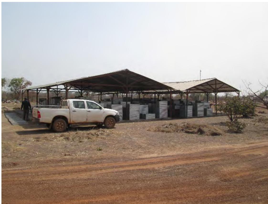
Figure 12.1 Shows the Core Storage and Logging Facilities at the New Camp
