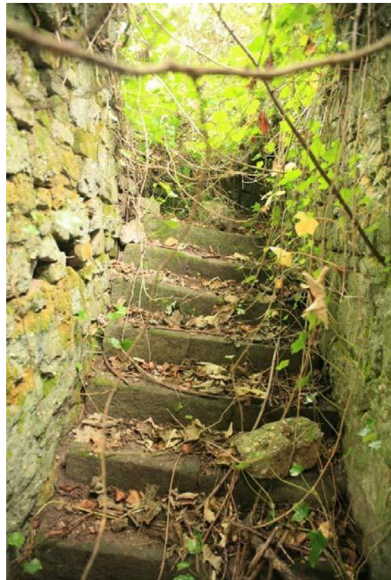
Fig.59 Footpaths are often enclosed to one or both sides by dry stone boundary walls and include important features such as stone steps
