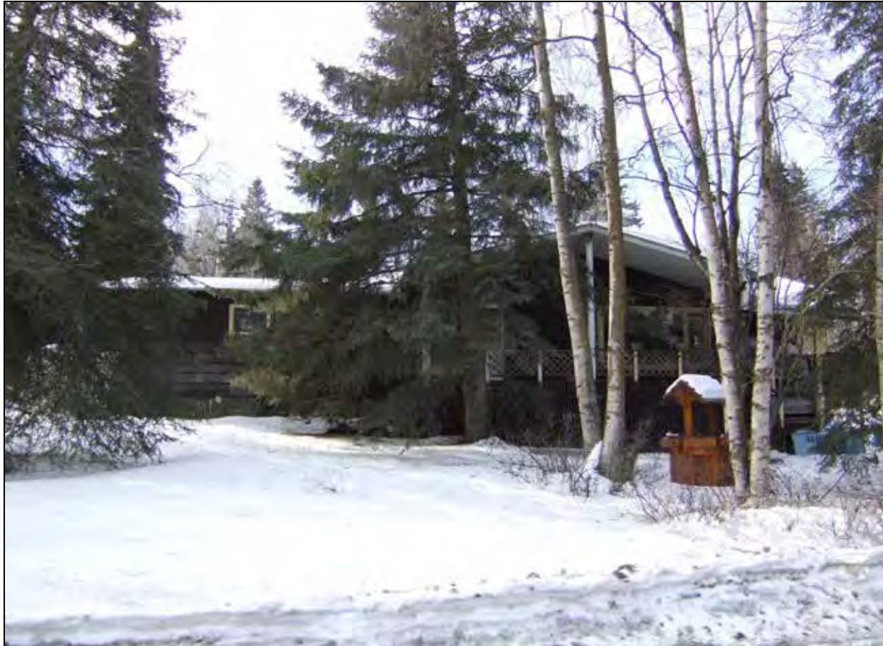
Site ANC-03468, 6014 Collins Way, Anchorage, Alaska Northeast façade, overview (Jewel Lake Rd 3-16-2011/029)
