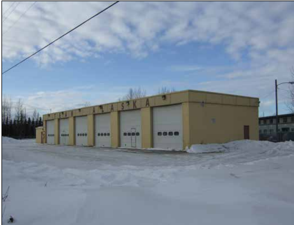
Site ANC003464, Alaska National Guard Vehicle Maintenance 4902 Spenard Road, Anchorage Alaska Northeast façade (Jewel Lake Rd 3-16-2011/007)
