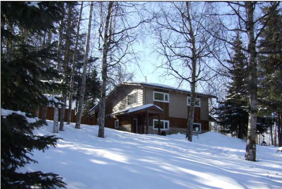
Figure 7.29. Overview of north and east façades of 3838 W. 63 rd Avenue, view to southwest.
