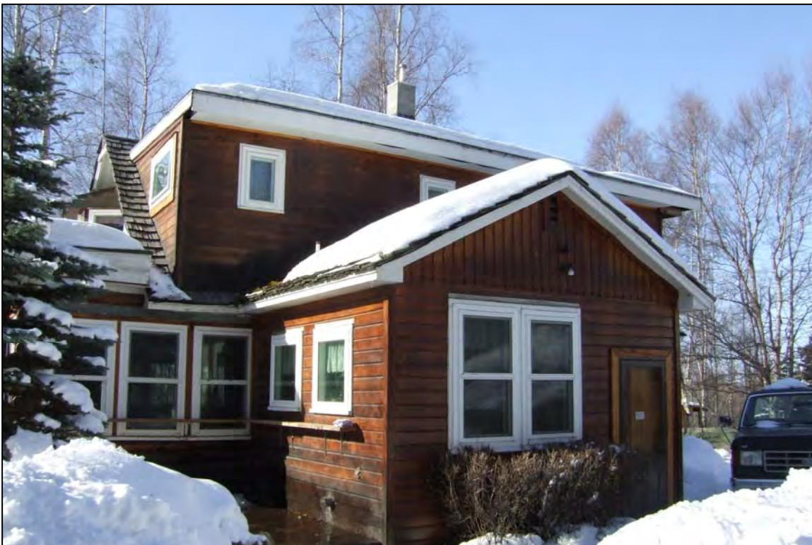
Figure 7.17. Central portion of east façade of 6141 Jewel Lake Road, view to northwest.
