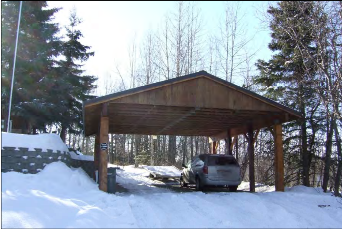
Figure 7.32. Front façade and interior of detached carport, 3838 W. 63 rd Avenue, view to south-southwest.
