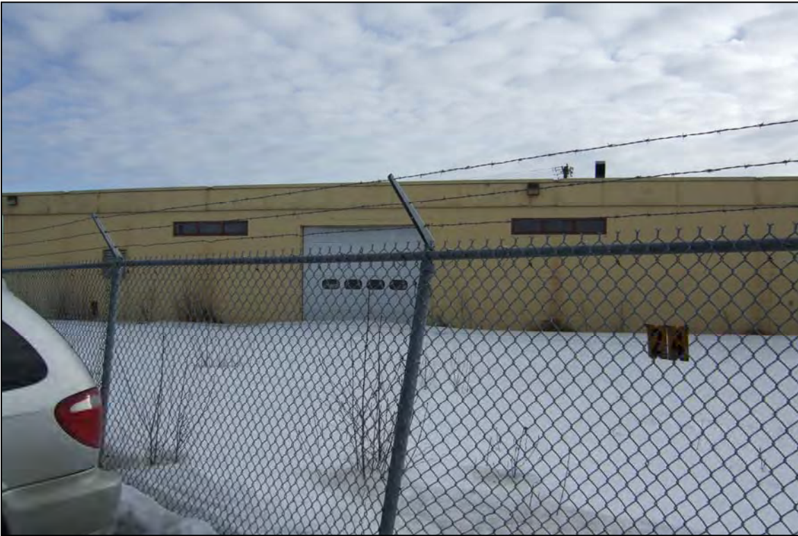
Figure 7.7. Central portion of southwest façade of 4902 Spenard Road, National Guard Vehicle Maintenance Building, view to northeast.
