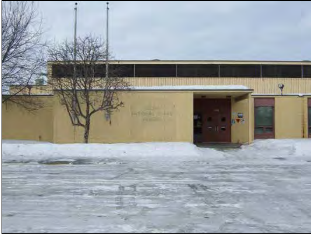
Site ANC-03463, Alaska National Guard Armory 4902 Spenard Road, Anchorage, Alaska Northeast façade, entrance overview (Jewel Lake Rd 3-16-2011/011)
