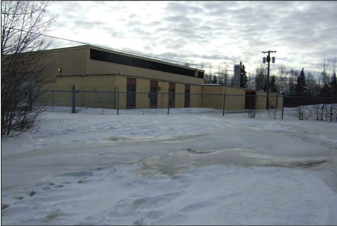
Figure 7.4. Overview of rear (southwest) façade of 4902 Spenard Road, National Guard Armory, view to south-southeast.
