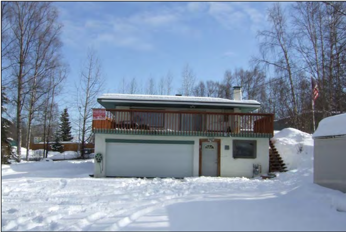
Figure 7.12. Overview of southwest façade of 3708 Jewel Lake Road, view to northeast.
