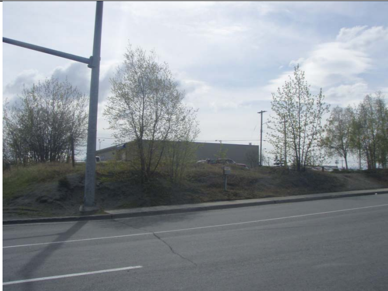
Facing South, Intersection of 3 rd Ave. and Ingra St. where rumble strips and restriping are proposed.
