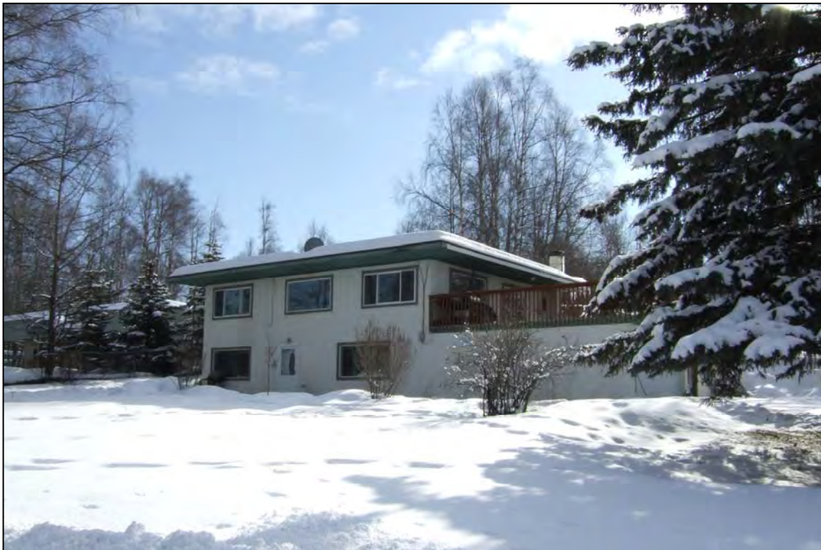
Figure 7.13. Overview of northwest façade of 3708 Jewel Lake Road, view to east.
