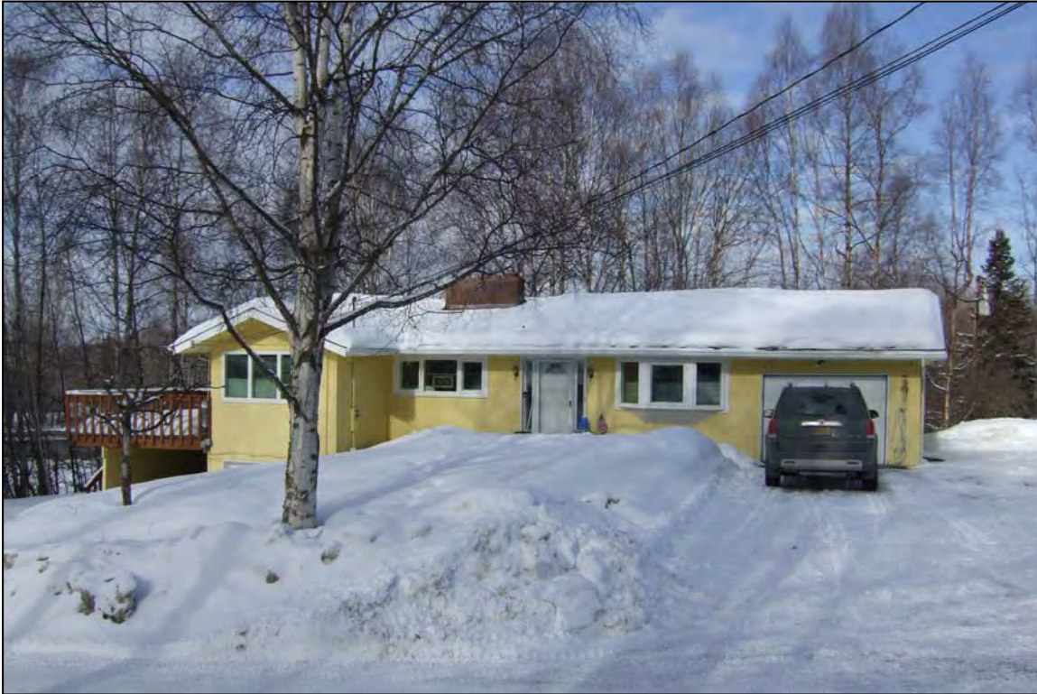
Figure 7.24. Overview of south façade of 3729 W. 61 st Avenue, view to north.
