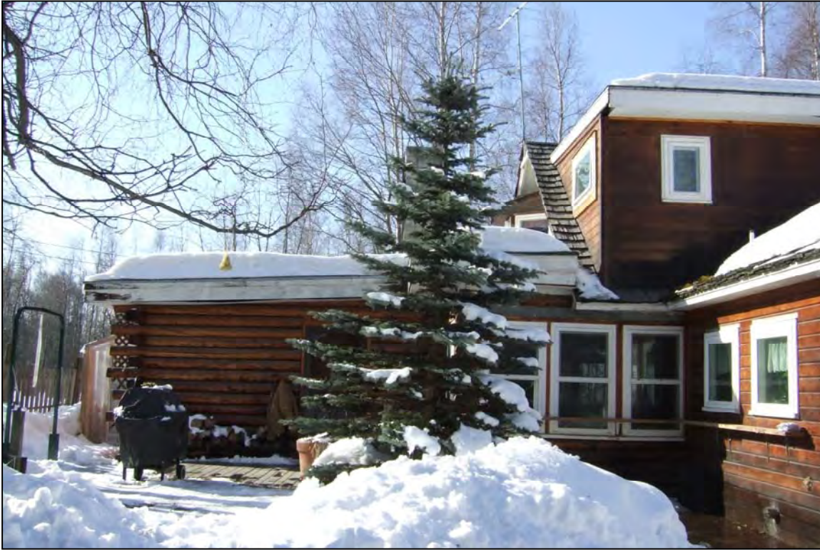
Figure 7.18. Southern portion of east façade of 6141 Jewel Lake Road, view to west.
