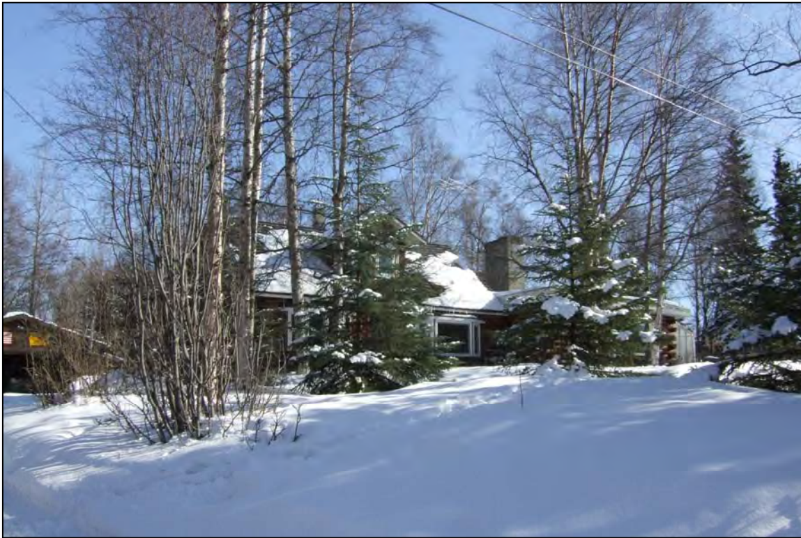
Figure 7.14. Overview of west façade of 6141 Jewel Lake Road, view to east-southeast.
