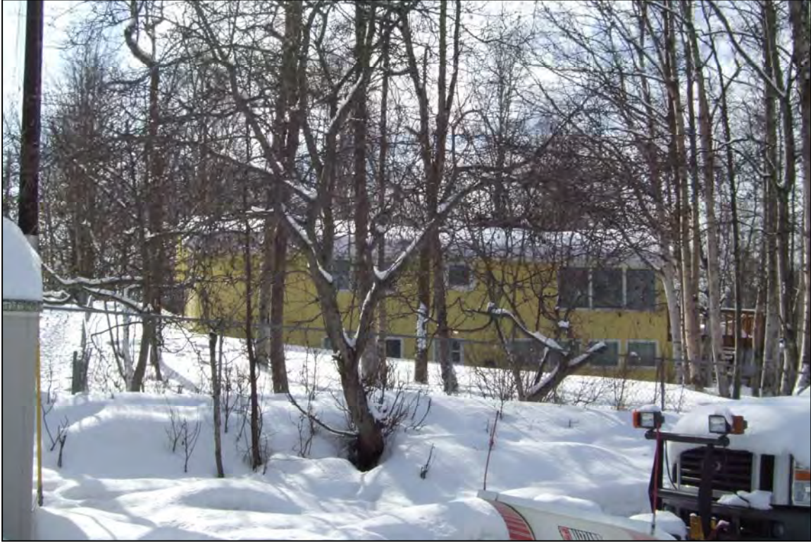
Figure 7.26. Overview of north façade of 3729 W. 61 st Avenue, view to south.
