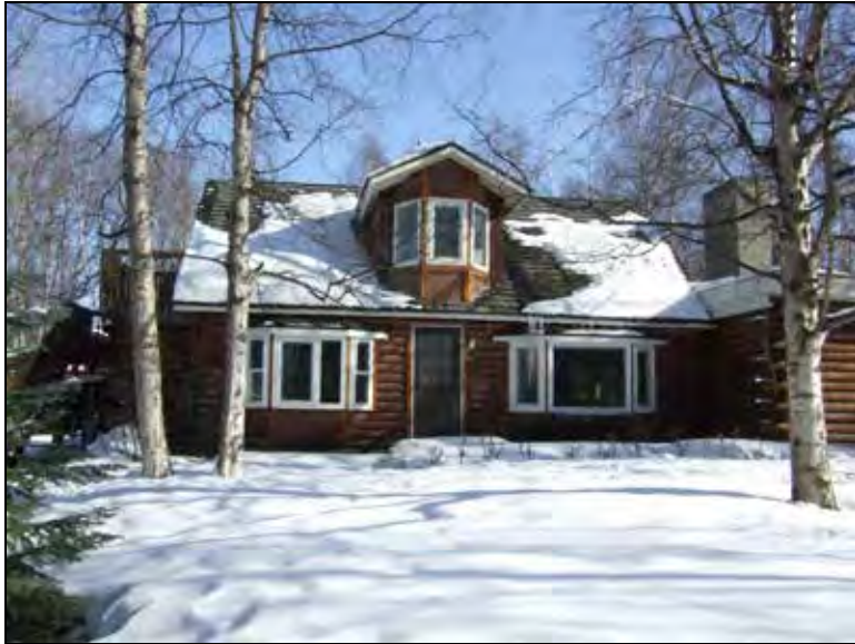
Site ANC-03467, 6141 Jewel Lake Road, Anchorage, Alaska West (front) façade, overview – north two-thirds (Jewel Lake Rd 3-19-2011/002)
