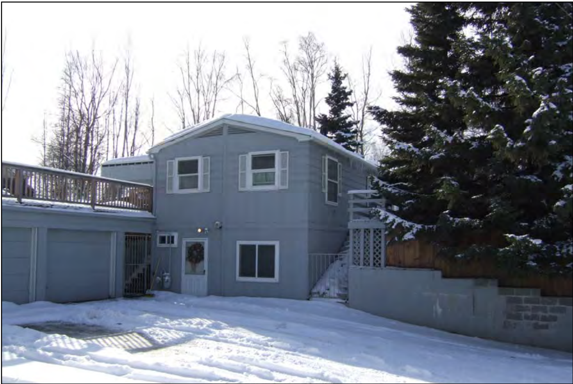
Figure 7.27. Overview of northeast façade of 3808 W. 61 st Avenue, view to south-southwest.
