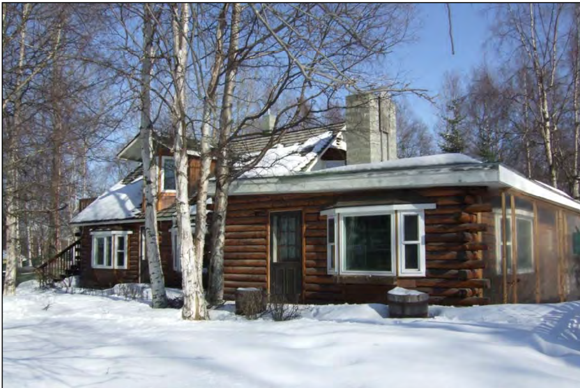
Figure 7.15. West and south façades of 6141 Jewel Lake Road, view to northeast.
