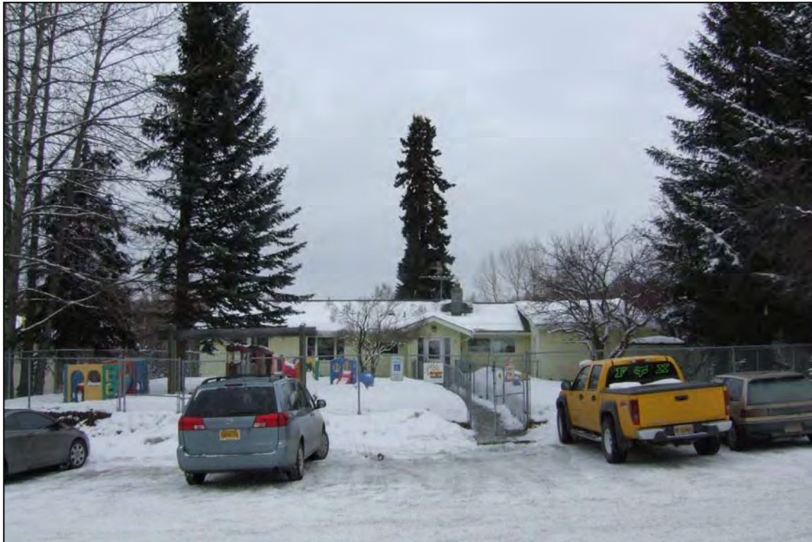
Figure 7.9. Overview of south façade of 3606 Jewel Lake Road, Bright Beginnings Early Learning Center, view to north.
