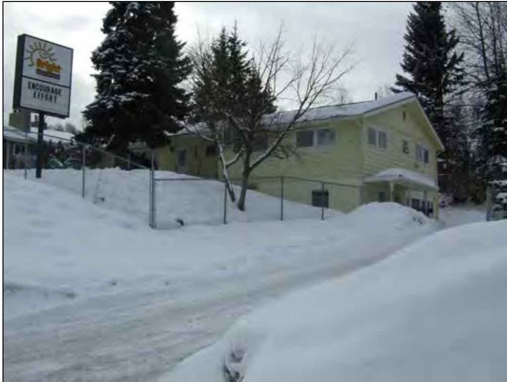
Site ANC-03465, 3606 Jewel Lake Road, Anchorage, Alaska West two-thirds of North façade (Jewel Lake Rd 3-18-2011/020)
