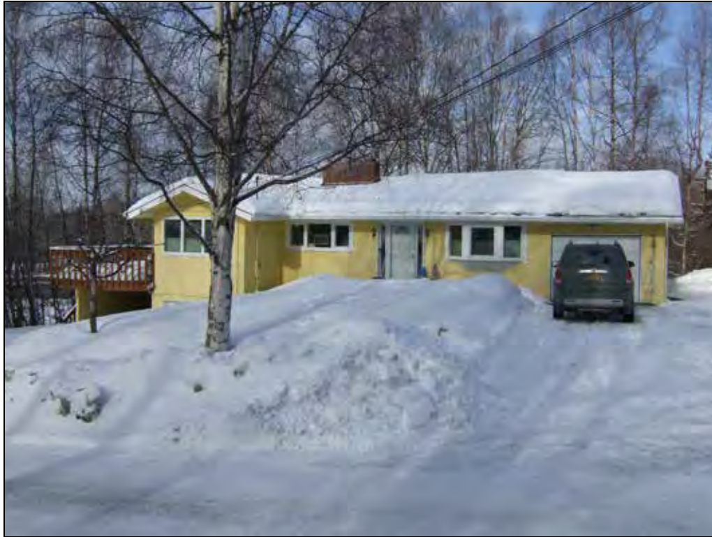
Site ANC-03469, 3729 W. 61 st Avenue, Anchorage, Alaska South (front) façade, overview (Jewel Lake Rd 3-18-2011/039)
