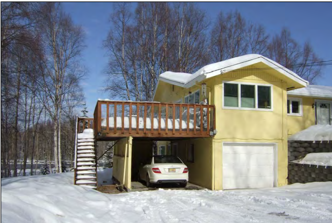
Figure 7.25. Overview of west and south façades of 3729 W. 61 st Avenue, view to northeast.
