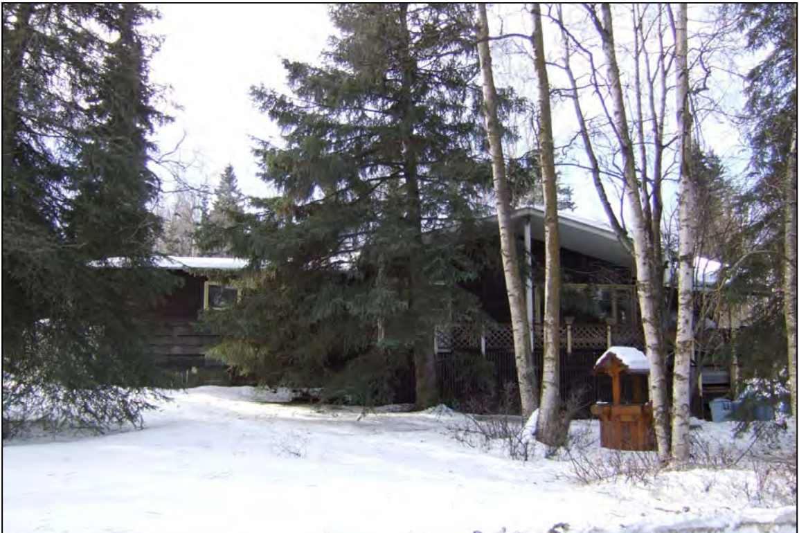
Figure 7.21. Overview of northeast façade of 6014 Collins Way, view to southwest.
