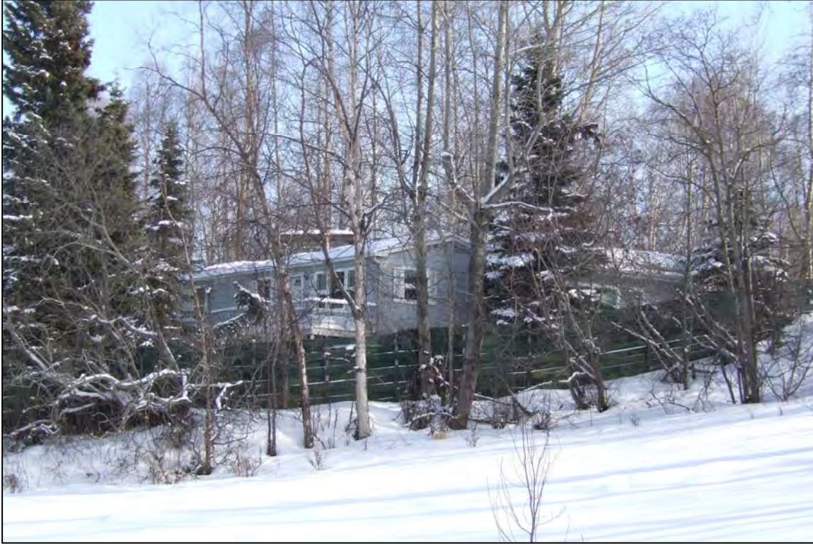
Figure 7.28. Overview of southeast and southwest façades of 3808 W. 61 st Avenue, view to northwest.
