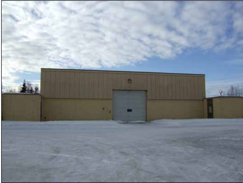
Site ANC-03463, Alaska National Guard Armory 4902 Spenard Road, Anchorage, Alaska Northwest façade, center (Jewel Lake Rd 3-16-2011/004)
