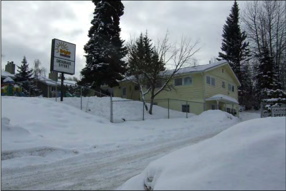
Figure 7.8. Overview of north façade of 3606 Jewel Lake Road, Bright Beginnings Early Learning Center, view to southeast.
