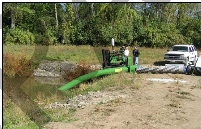
Photograph 5-5. Portable Pump-Lake Odessa HREP, Pools 17-18, UMR RM 435.0-440.0, Louisa Co., IA, MVR
