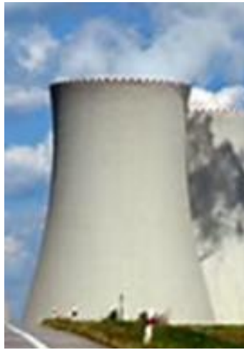
Fig. 1 – Typical water cooling tower.
