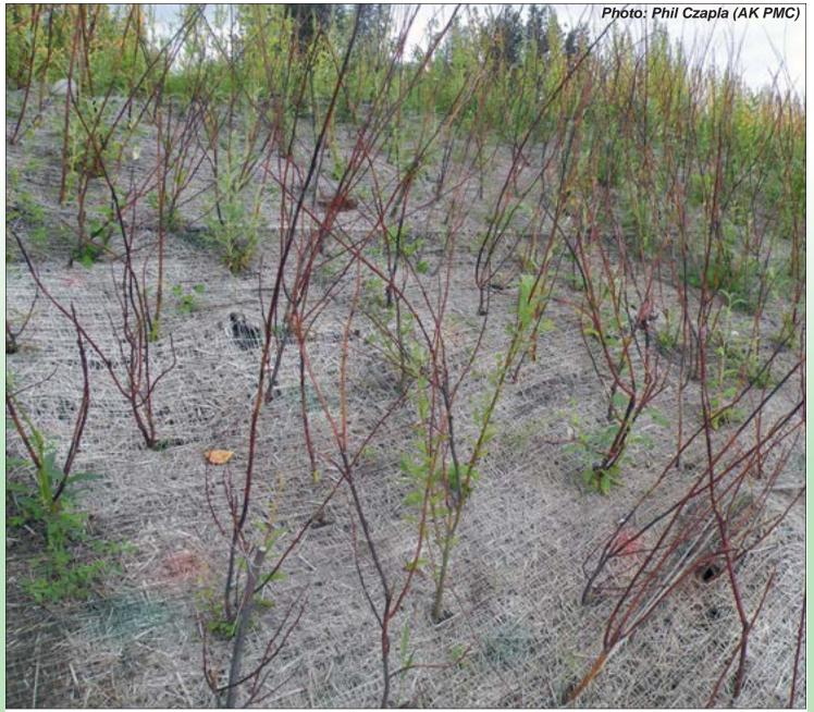
Figure 19: Erosion Control matting can stabilize a cut slope while seed or transplants become established
