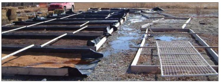
10' x 3' constructed mats framed with dimensional lumber, with thick plastic and erosion control matting used for the base. Only the biodegradable erosion control matting will remain once the mat is deployed.
