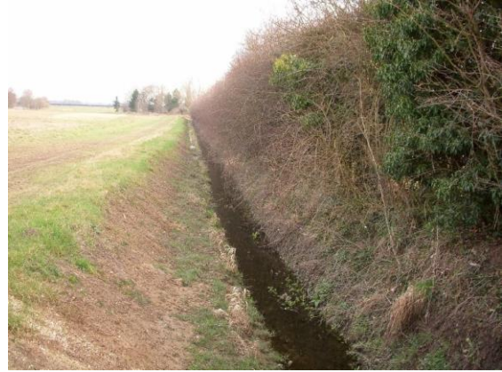
Plate 4 Restored ditch to give two-stage channel.
