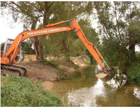
Plate 2 Shoal creation through gravel placement
