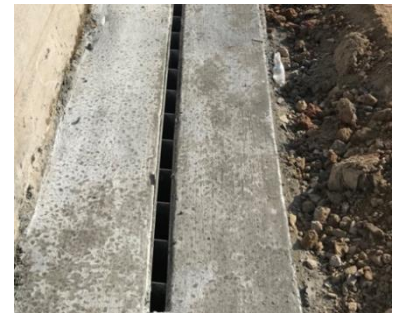
Completed Duraslot Installation
