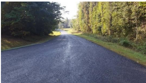
Roadway recently treated with Fog Seal
