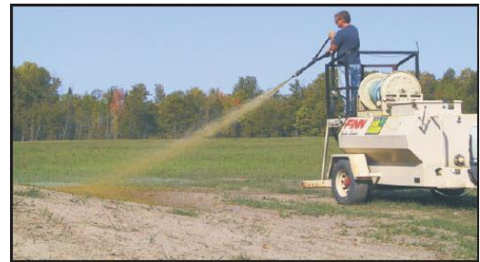
Example of Flex Guard being applied – image from Mat, Inc. website
