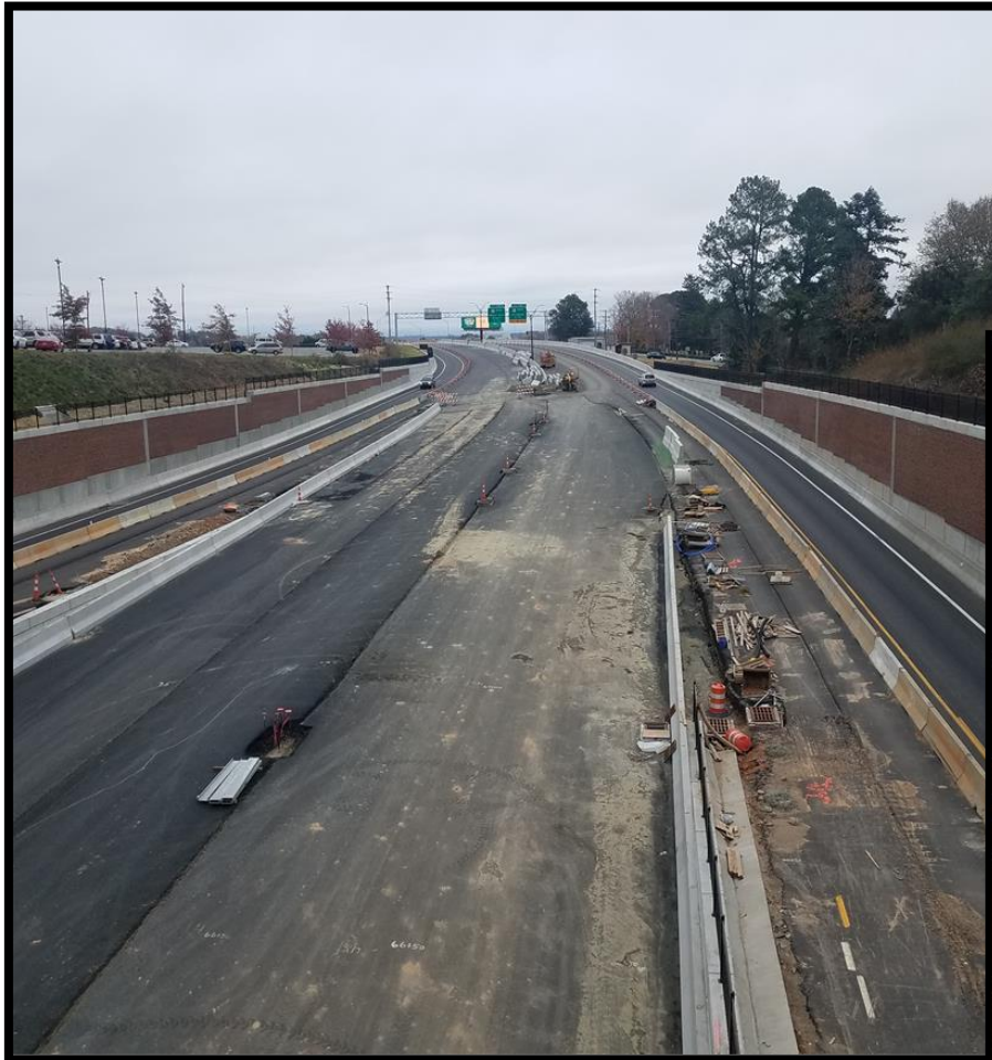
Salem Parkway looking east from Church Street
