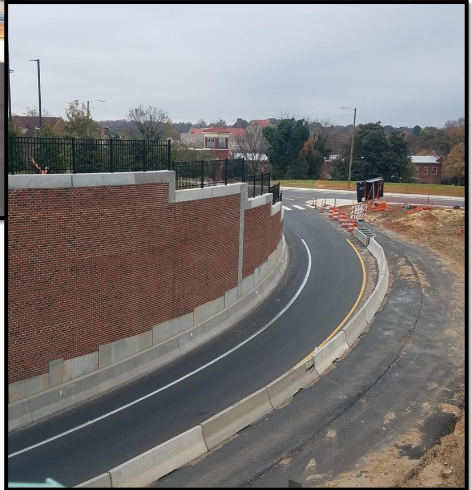
Retaining wall with brick enhancements and decorative railing
