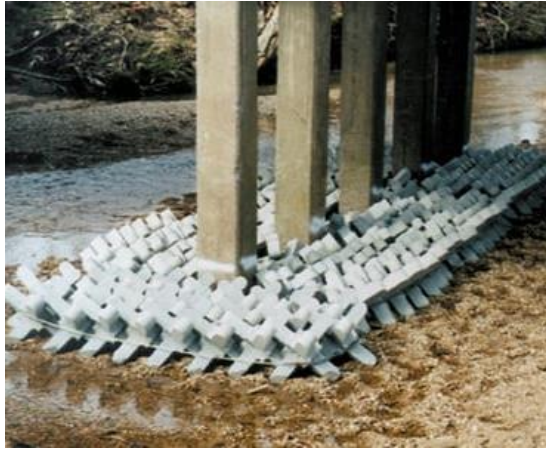
Example of A-Jacks installed for bridge scour protection – image from Contech website
