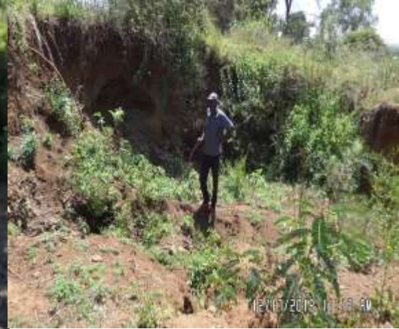
Figure 7-2: Derelict quarry land (MS 205) susceptible to landslide
