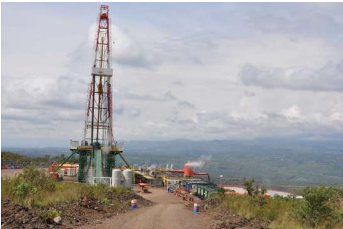
Figure 2-4: Drilling Rig at Menengai, Kenya (source: ARGeo)
