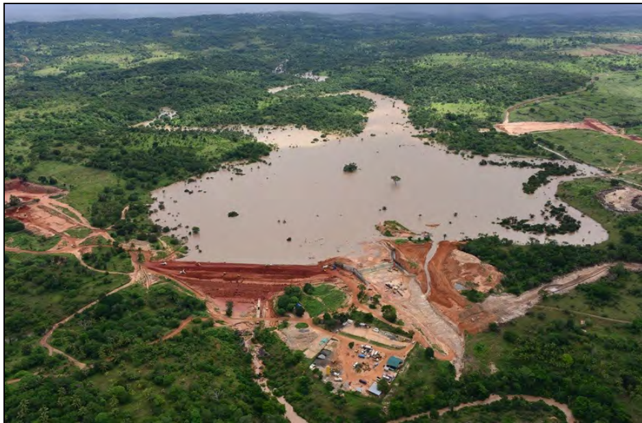
(Base Mkurumudzi Dam – under construction)
