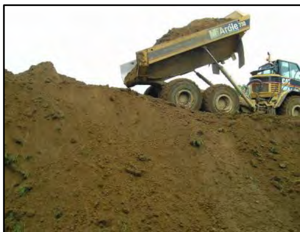
Figure 24. Stockpiling topsoil.
