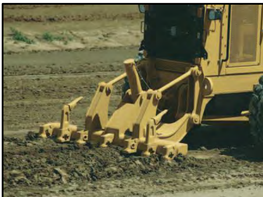
Figure 26: Grader ripping compacted soil.
