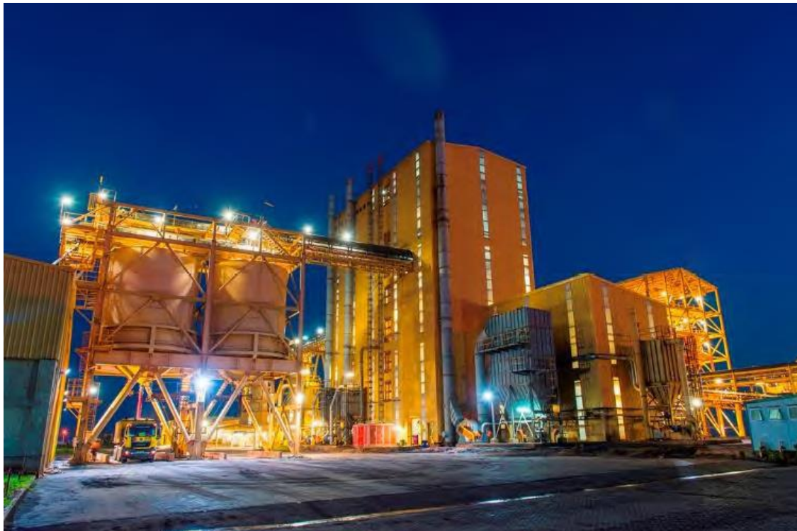
Figure 2.5: The Kwale Mineral Sands Mineral Separation Plant (MSP).
