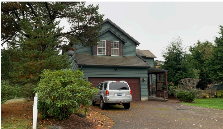
Exhibit 160. Example of Newport Medium Single-Detached House Source: ECONorthwest
