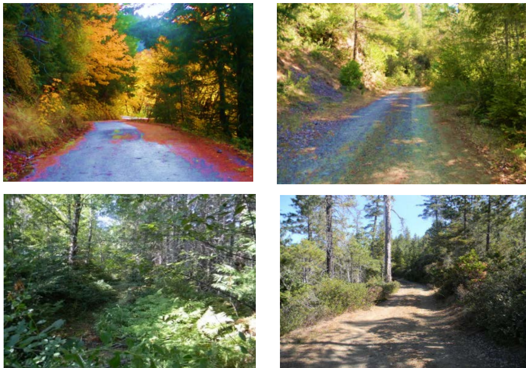
Figure 1-1. Photos (clockwise from upper left): ML 3 road designed for highway-legal passenger cars; ML 2 road designed for high-clearance wheeled vehicles; UAR used as a motorized trail; and, ML 1 road in storage.
