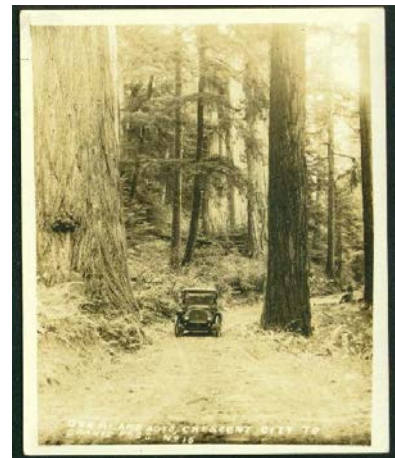
Figure 1-3. Howland Hills Road used to haul logs out of what is now the Smith River NRA.
