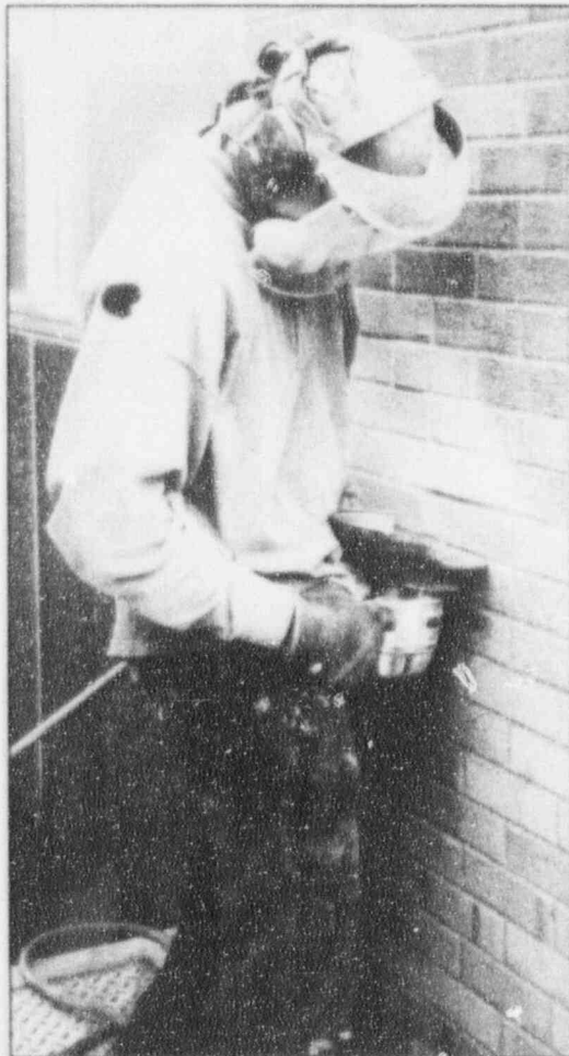
Left, an employee of Karr Tuckpointing, Vinton, repairs crumbled mortar outside Corn Belt Power's headquarters building.
