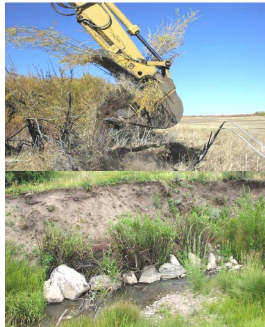
Figure 3. Willow clumps being removed from a local stand (above) and established willow clumps in a riparian planting (below). Chris Hoag, NRCS.
