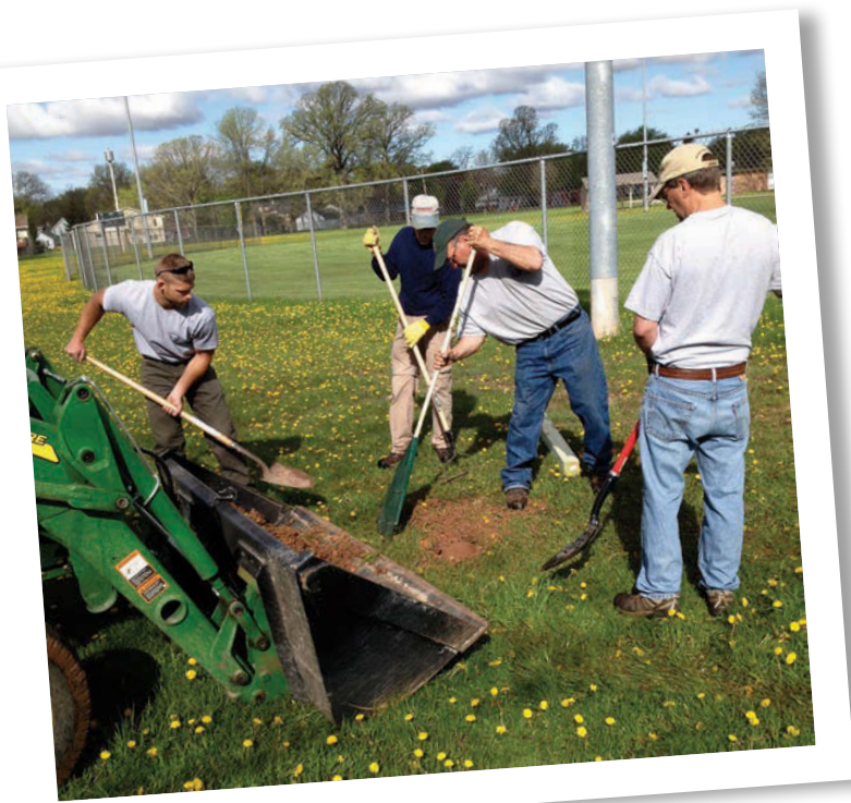
I shot this photo with my iPhone of some work being done in a local park in my hometown this summer. Photos taken with the latest generation of smartphones can provide quality documentation of your installation work.
