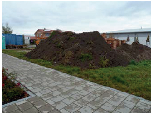
Fig 10: Excavated soil at the construction site „Am Falkenhorst“ in Hiltpoltstein.
