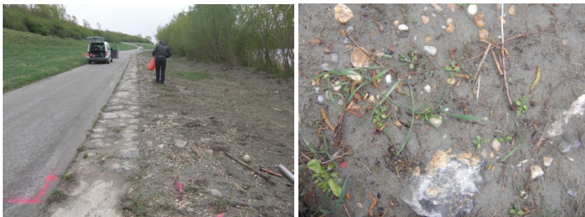
Fig. 4: Overview (left) and detail (right) of plot 4 along the river
