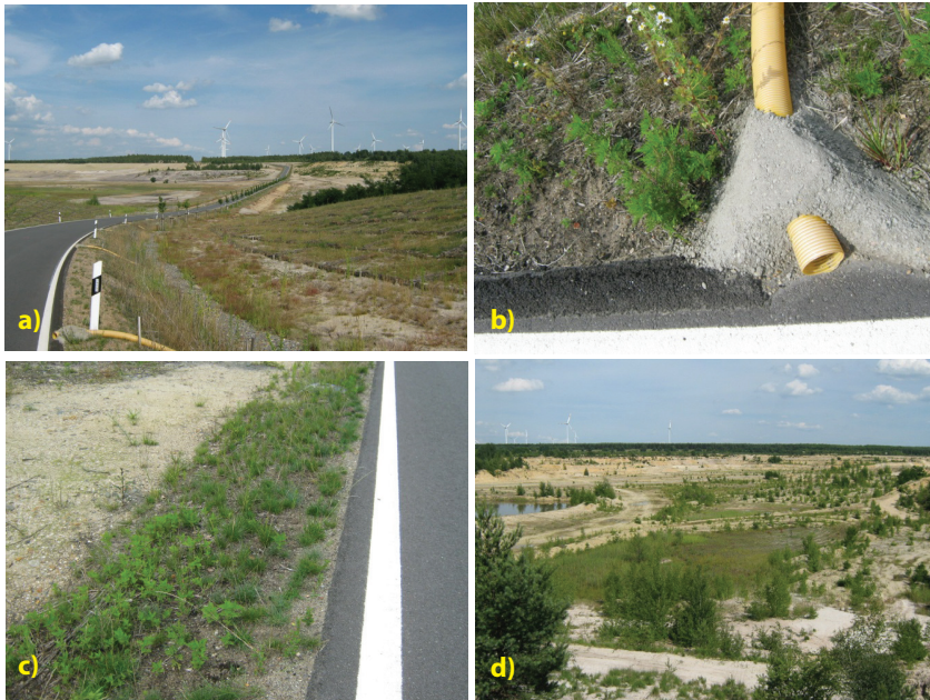
Fig 15: Newly built road in a reconstruction area connecting the villages Klettwitz and Kostebrau near Senftenberg (photo: 2011/07/06).
