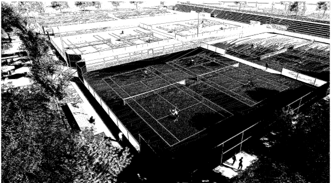
Figure 69: Zone B tennis courts
