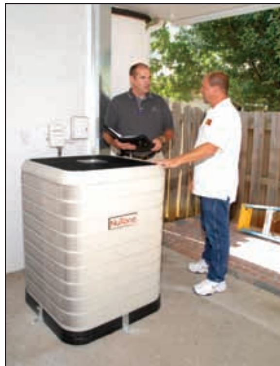
Steve Queen (left), manager of Noland Company in Longwood, Fla., and Craig Marcelle of Comfort Experts USA in Melbourne discuss the installation of NuTone Heating and Cooling Products air conditioner at a residence. The unit is rated 3-ton, 22 SEER with iQ Drive® technology. Comfort Experts is installing NuTone heat pump systems distributed by Noland in the Turtle Creek home development in Rockledge.
