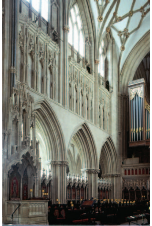
FIG. 4. Wells cathedral: choir, showing 12th-century arcades and 14th-century rebuilding above Malcolm Thurlby
