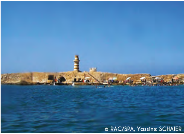
Figure 158. Northern inlet of Saida, an interesting place to be protected
