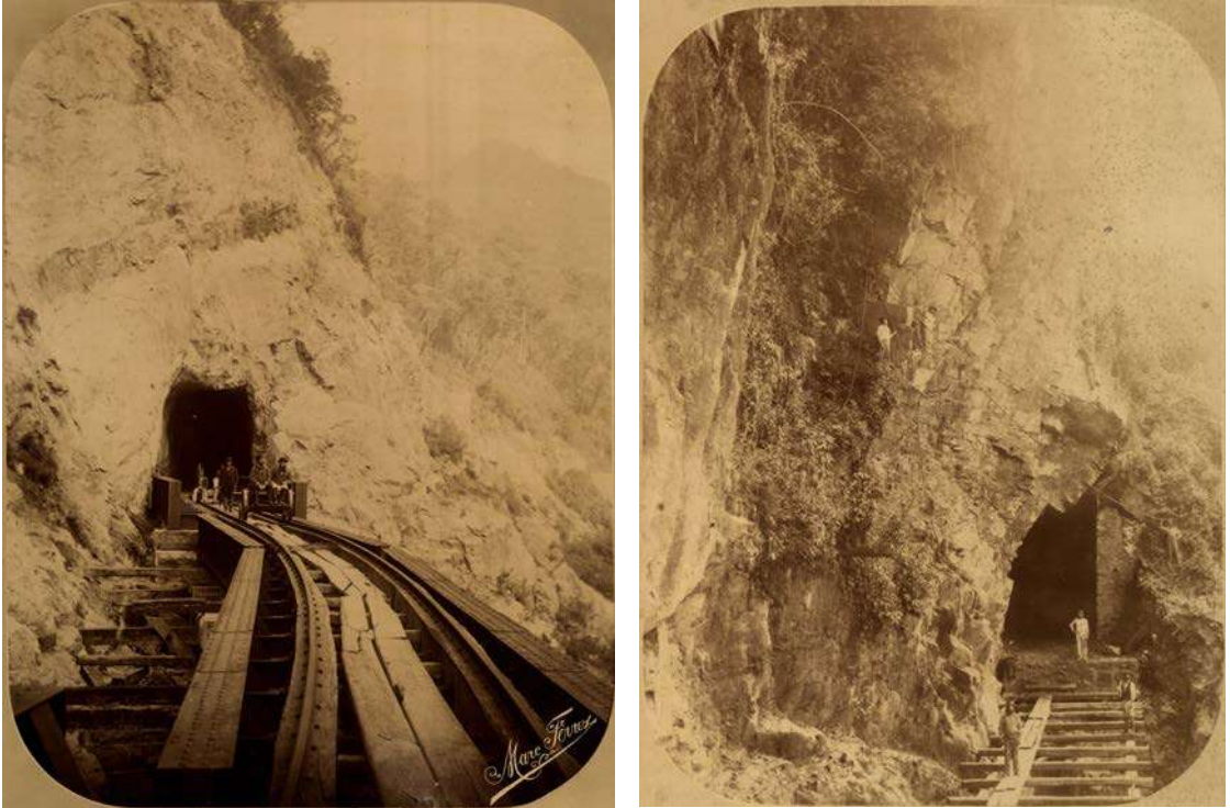
FIGURE 65. Parana Railway under construction, early 1880s. Photographs by Marc Ferrez.
