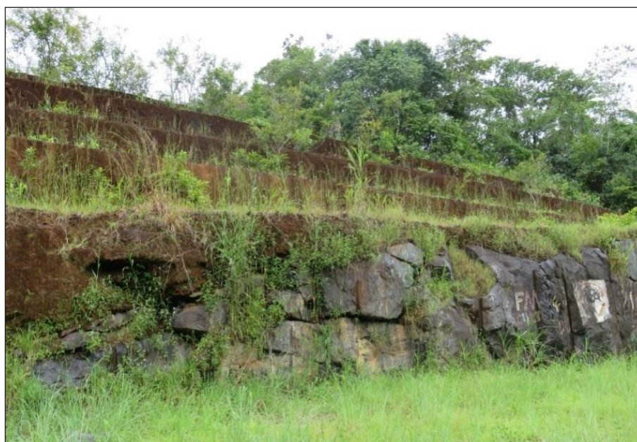
Figure C.7.9: Benched cut slope in residual soils above rock
