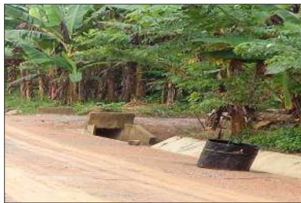
Figure C.4.10: Typical access culvert at a junction
