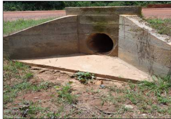
Figure C.6.5: Concrete apron at culvert outlet
