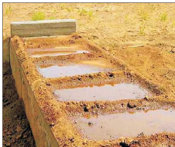
Figure C.8.7: Curing concrete slab by ponding
