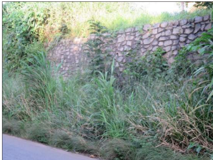
Figure C.7.16: Mortared masonry wall providing shallow support and slope protection
