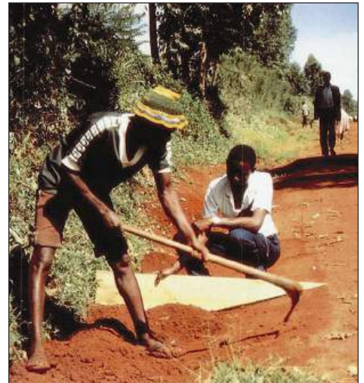
Figure C.9.5: Checking drain shape with template
