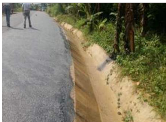
Figure C.4.2: Concrete lined trapezoidal drain
