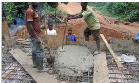
Figure C.8.14: Constructing reinforced concrete slab
