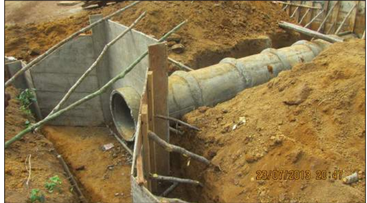
Figure C.6.2: Reinforced concrete pipe culvert
