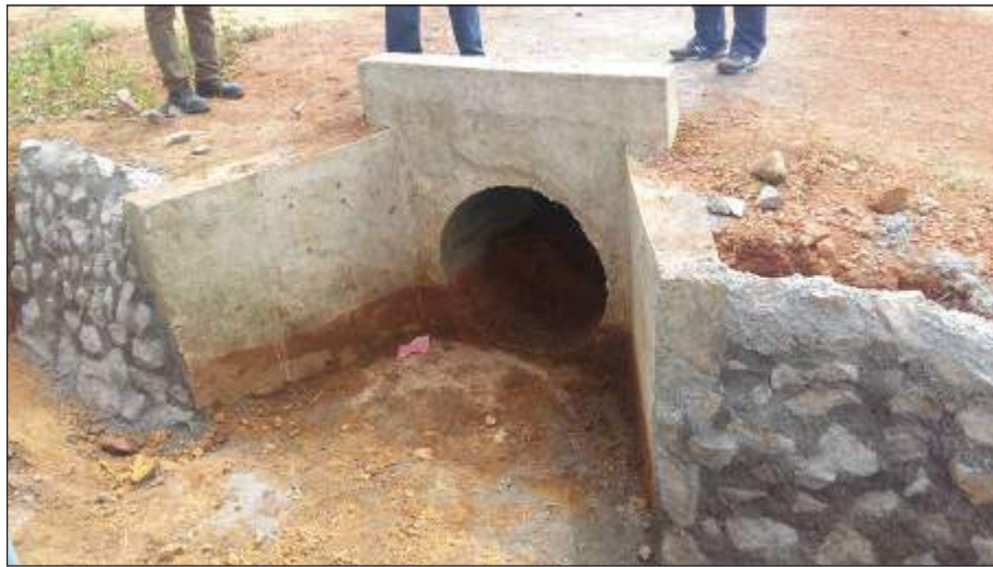
Figure C.8.15: Stone pitched embankment slopes behind wingwalls
