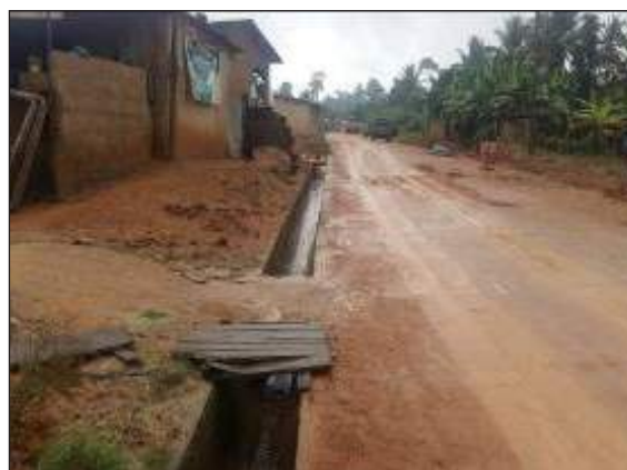
Figure C.4.3: Concrete lined U-drain
