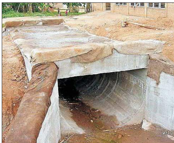
Figure C.8.6: Curing of concrete with wet hessian sacking
