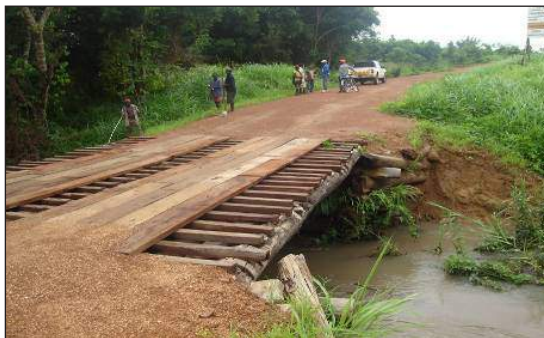
Figure C.8.19: Timber bridge deck
