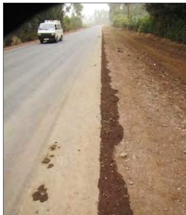
Figure C.2.4: Infiltration of water through a permeable surfacing
