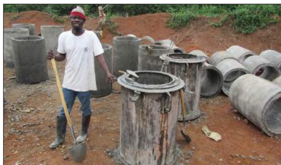
Figure C.8.13: Concrete culvert ring production
