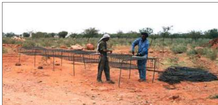
Figure C.8.4: Steel reinforcement cage being assembled
