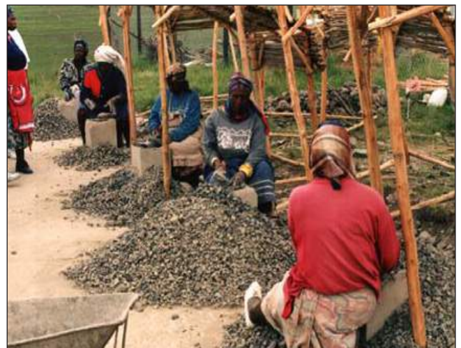
Figure C.8.3: Aggregate being crushed by hand
