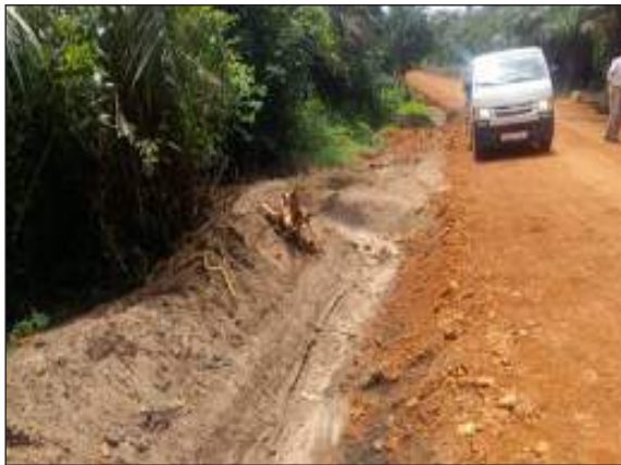
Figure C.4.4: Mitre drain on an LVR
