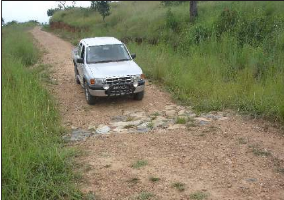
Figure C.4.14: Simple drift using hand packed stone
