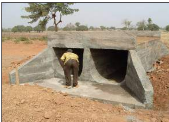
Figure C.4.9: Typical U-culvert
