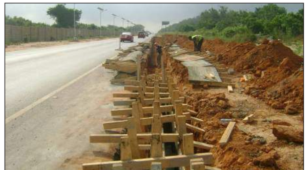
Figure C.8.20: Timber formwork
