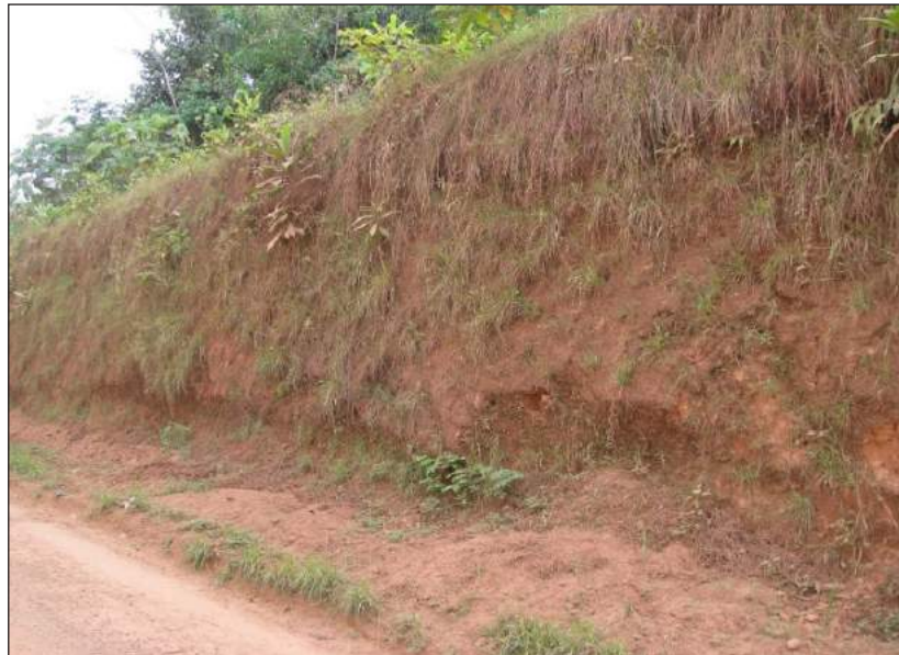
Figure C.7.7: Cut Slope in WG V-VI Material at 3V:1H and still intact after 40 years
