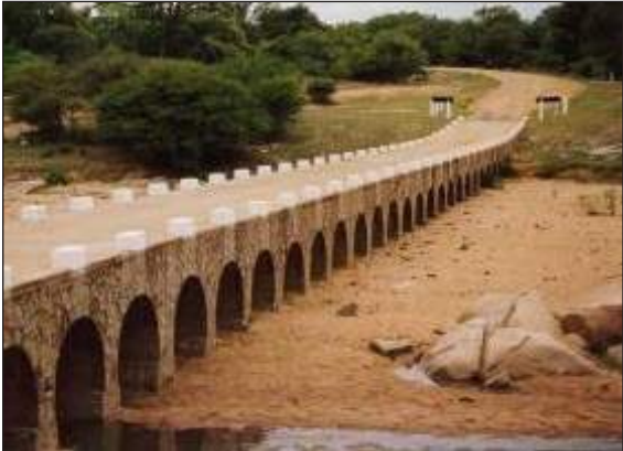
Figure C.4.13: Large vented drift
