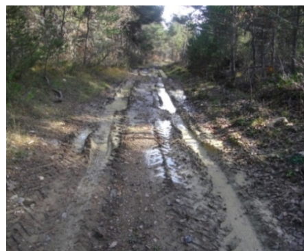
Figure 3. Example images of deformation on the road surface
