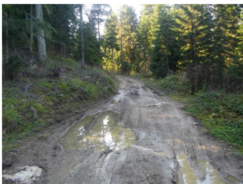
Figure 3. Example images of deformation on the road surface
