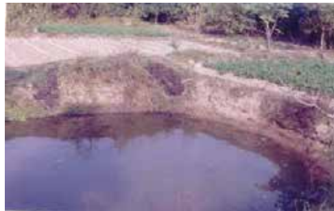
Plate 2 : Sub surface water harvesting structure at Erasam block, Odisha
