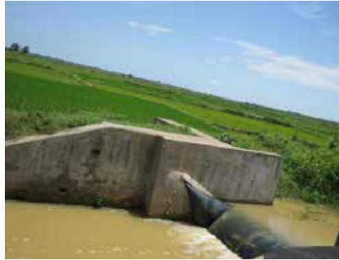
Plate1: Rubber dam with adjacent paddy fields at Chandeswar, Odisha
