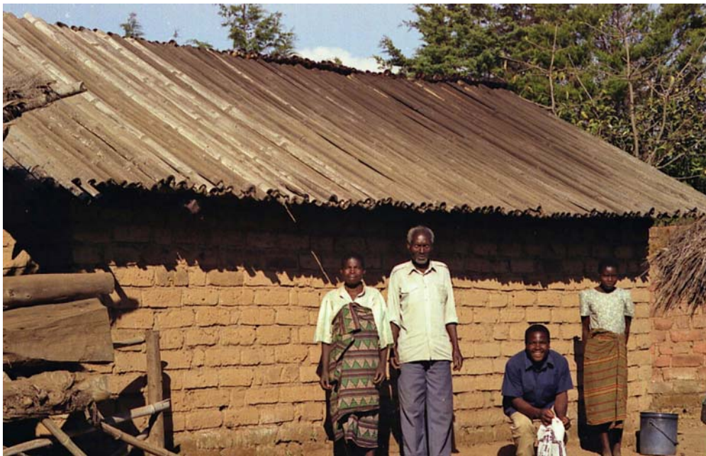
Matambo Salima with his family at Izumbwe. The house is roofed with split bamboo poles.
