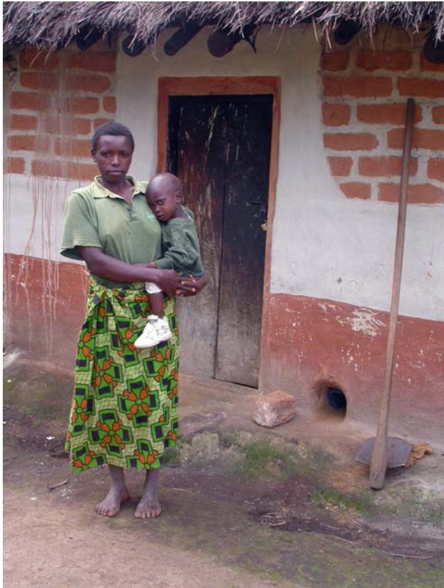
Many houses have a hole in the wall to allow chickens to come and go. The hole can be blocked off with a brick as necessary, to keep hens in until they have laid or to prevent snakes from entering.
