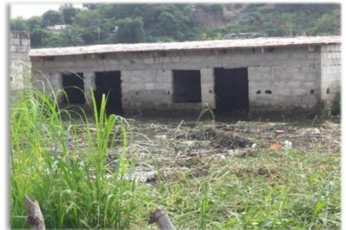
Figure 3: Flooding in district 9 Djiri
