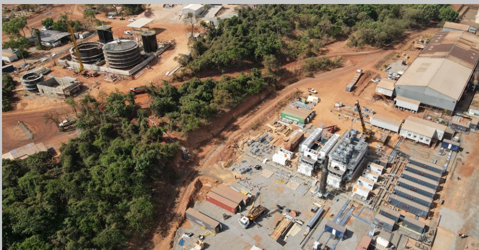
Syama Hybrid Power Station (right) & HFO Fuel Farm (left) construction areas
