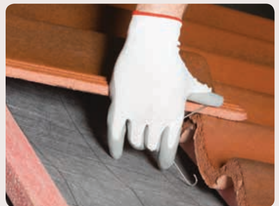
INNOFIX CLIP: A NEW WAY OF TILE FIXING FOR THE INDUSTRY
