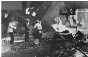
3-ton electric arc furnace at the time of establishment (1933)
