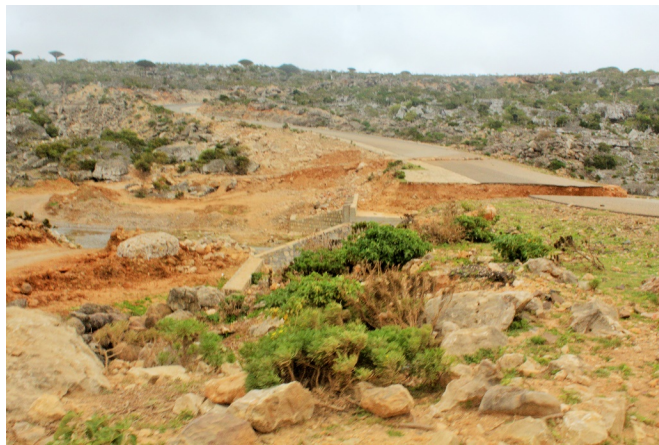
Figure 10. Road construction endangering ecosystem (photo by author, Socotra 2018).
