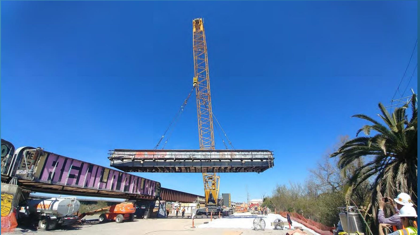
San Diego River Bridge Demolition
