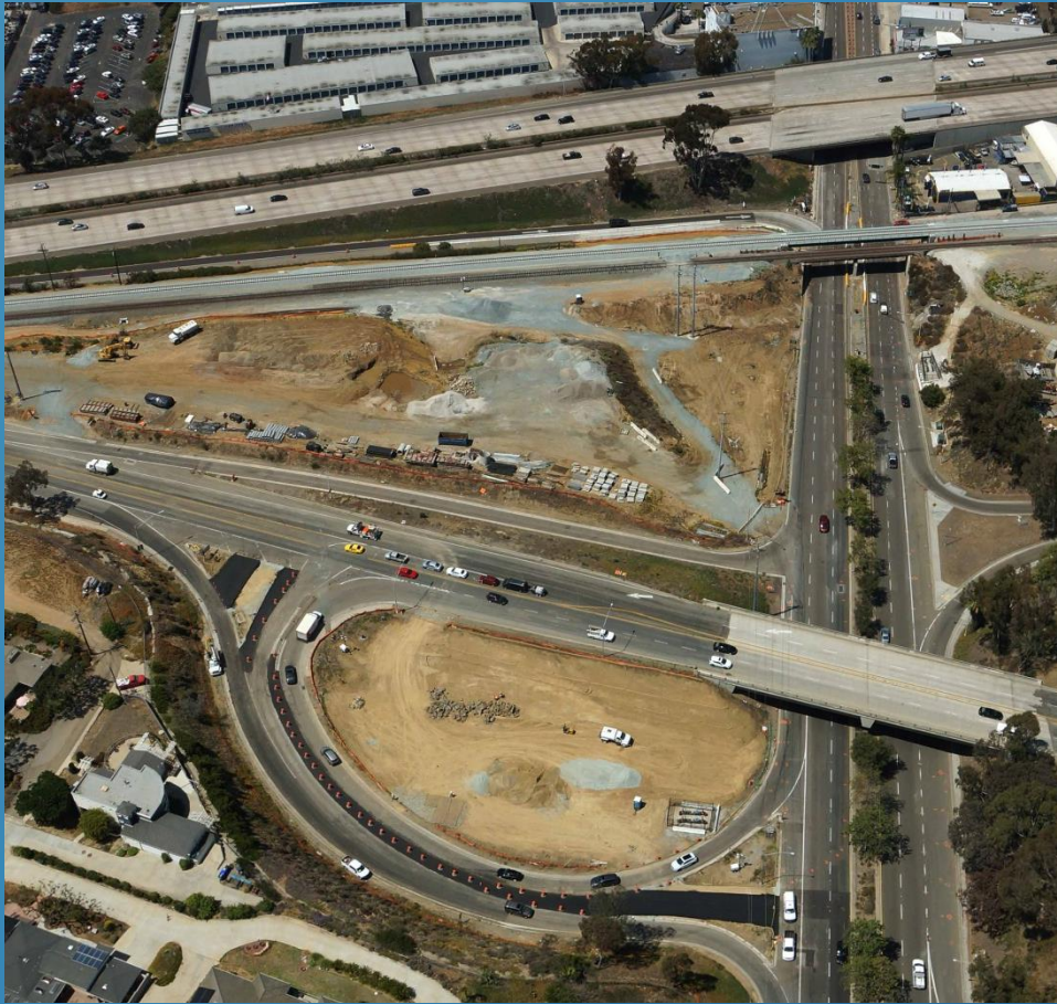
Future Balboa Avenue Station Site
