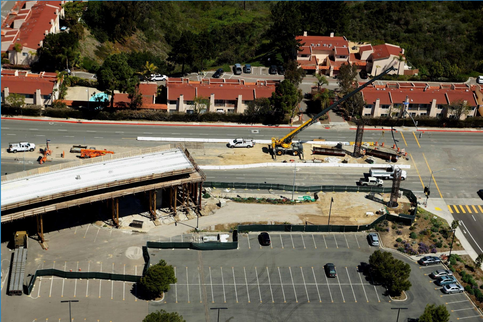
End of UC San Diego Viaduct – Beginning of Genesee Viaduct
