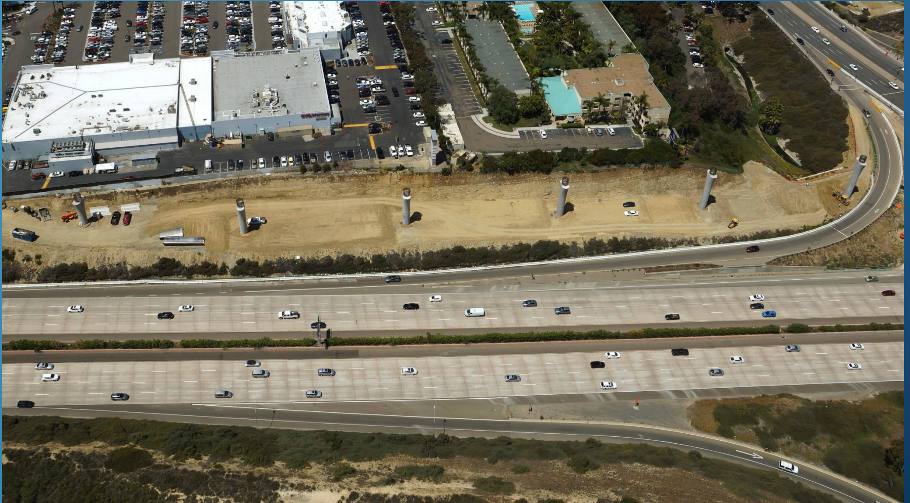
Nobel Viaduct – north of Nobel Drive
