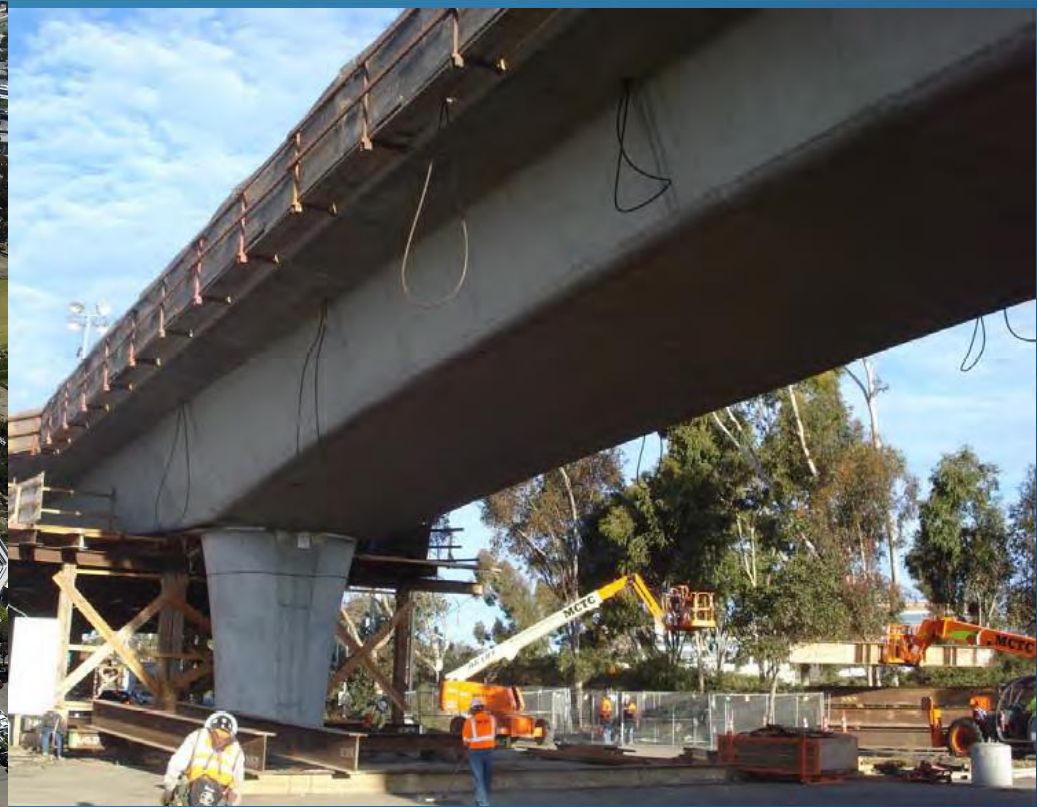
UC San Diego Viaduct – Removing Falsework
