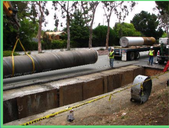
Utilities and Roads
