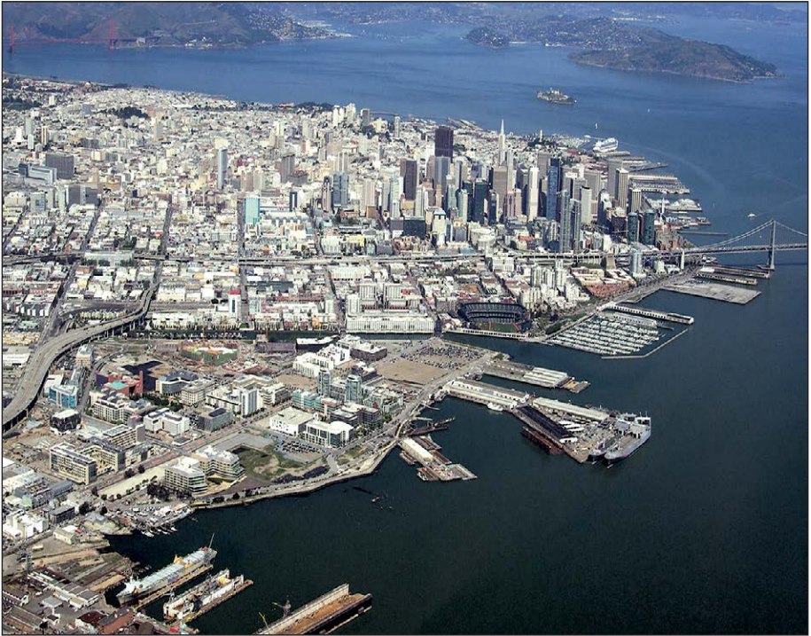
Photo courtesy of the Port of San Francisco
