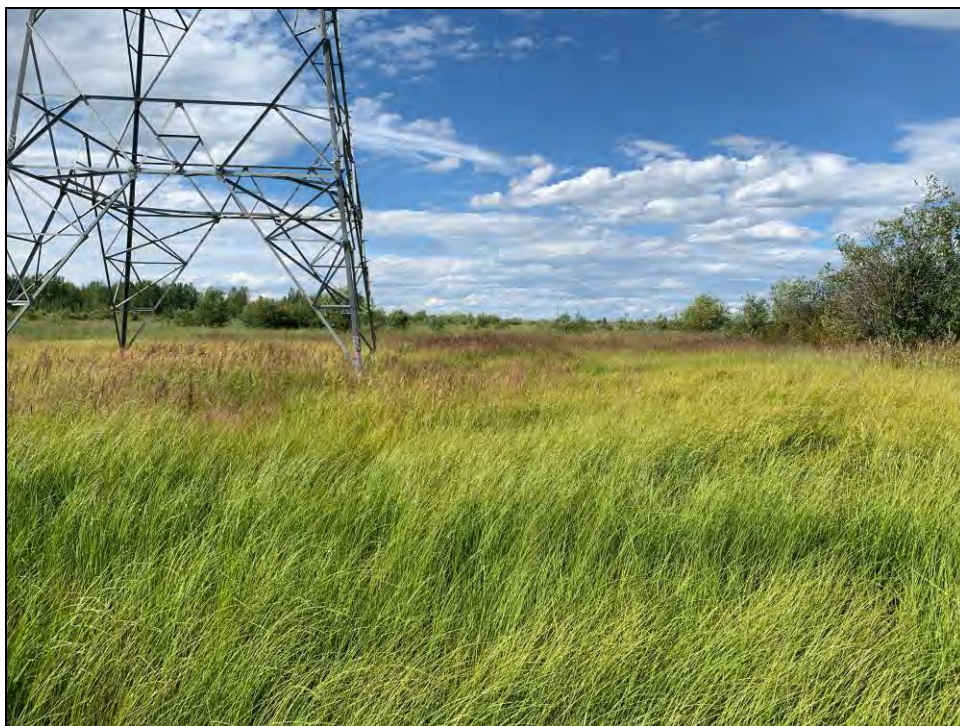
Plate 3.3-7. Wm00 Unclassified marsh at OWL021 in a modified area at the base of a new transmission line tower.
