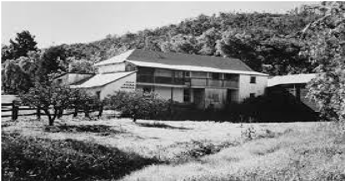
Figure 7-2 Whitby Falls Hostel (Conservation Plan, Griffiths Architects 2013)
