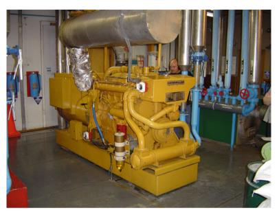
Fig. 26.6 One of three 225 kVA Caterpillar diesel generators at New Zealand's Scott Base (© Pat Bodger)
