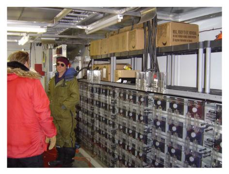
Fig. 26.2 The battery bank at the Mount Newell field station with 36 sealed lead-calcium batteries (© Pat Bodger)
