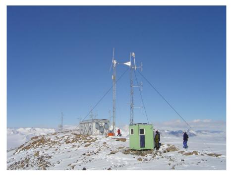
Fig. 26.5 These images show a portable wind generator which has been set up at to supply electricity for the operation of communications equipment (© Pat Bodger)
