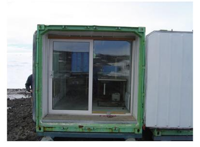
Fig. 26.4 This shipping container has been converted into a portable scientific laboratory ( $\[mathbb{C}\]$  Pat Bodger)
