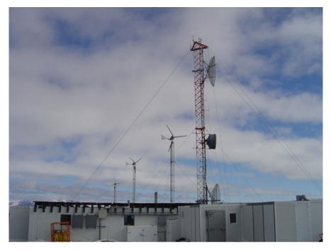
Fig. 26.1 The power-generation equipment at the Mount Newell field station consists of one diesel-fuelled generator, a solar array and a wind generator (© Pat Bodger)
