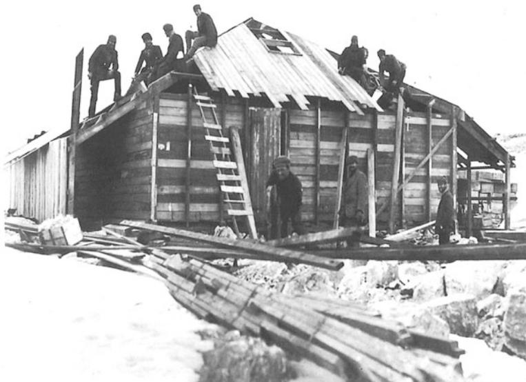
**Fig. 15.6** Erecting the hut at Commonwealth Bay. The huts were often pre-fabricated like a modular home (Reprinted from Martin 1996)
