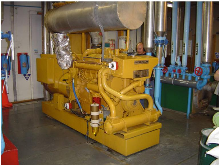
**Fig. 26.6** One of three 225 kVA Caterpillar diesel generators at New Zealand's Scott Base (© Pat Bodger)
