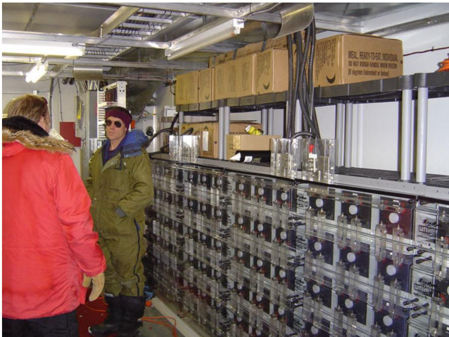
**Fig. 26.2** The battery bank at the Mount Newell field station with 36 sealed lead-calcium batteries
