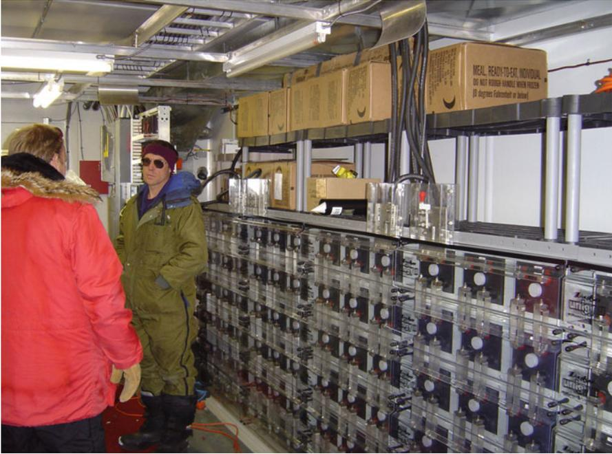
**Fig. 26.2** The battery bank at the Mount Newell field station with 36 sealed lead-calcium batteries (© Pat Bodger)
