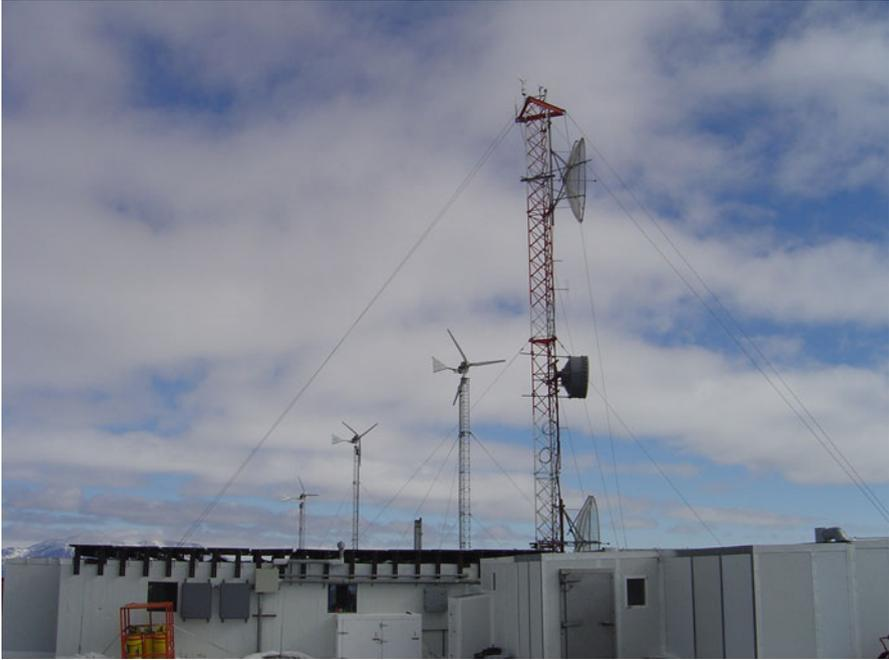
**Fig. 26.1** The power-generation equipment at the Mount Newell field station consists of one diesel-fuelled generator, a solar array and a wind generator (© Pat Bodger)
