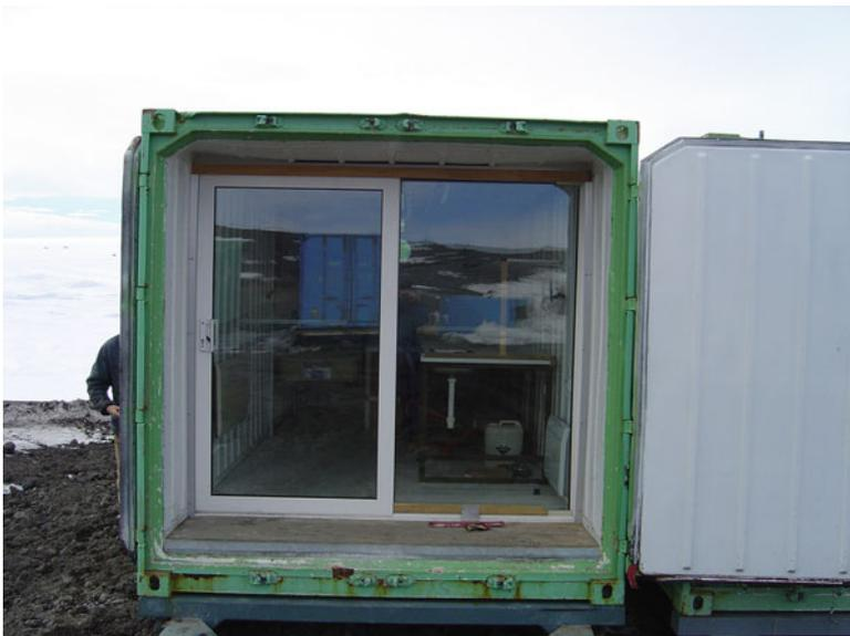
Fig. 26.4 This shipping container has been converted into a portable scientific laboratory (© Pat Bodger)
