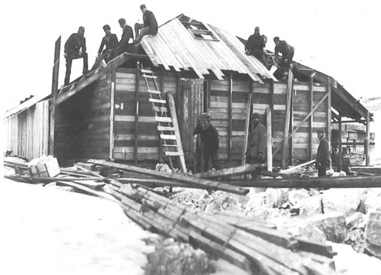
**Fig. 15.6** Erecting the hut at Commonwealth Bay. The huts were often pre-fabricated like a modular home (Reprinted from Martin 1996)
