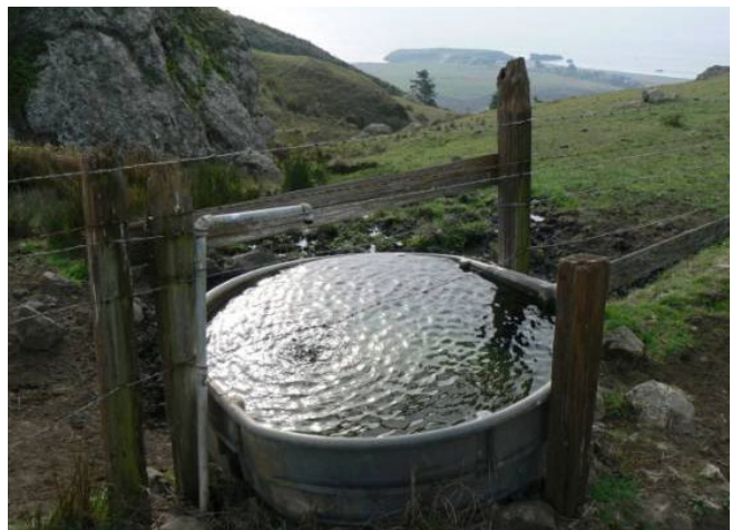
Water tank for house (top) and developed spring for livestock (bottom).
