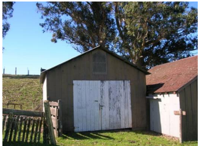
Garage (top) and shed (bottom) on Wright Hill Ranch.
