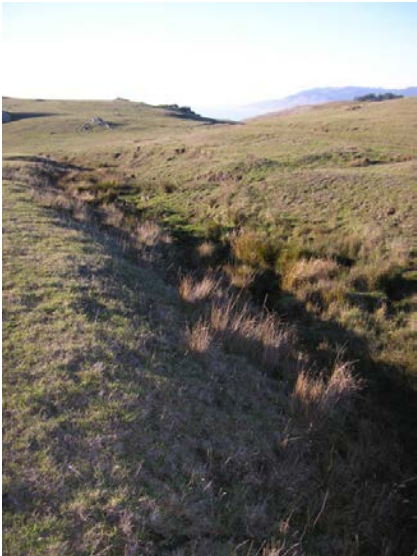
Photopoint 91. Headcut of Furlong Gulch looking downslope.
