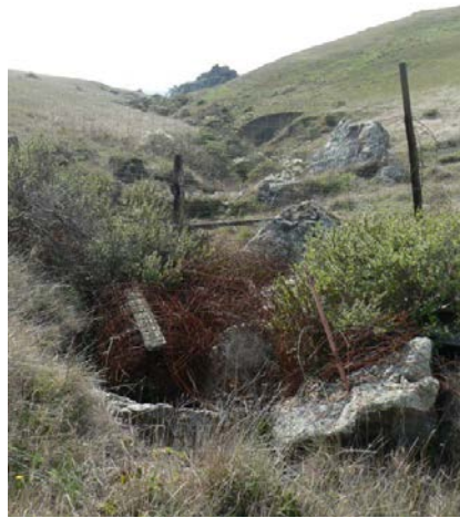
Photopoint 6. Gully 1 at property line
