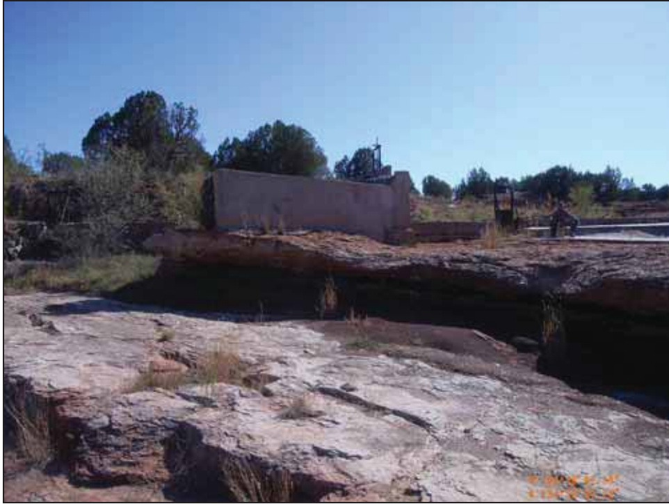
Figure 4.40. View of headgate and gabion, facing south.
