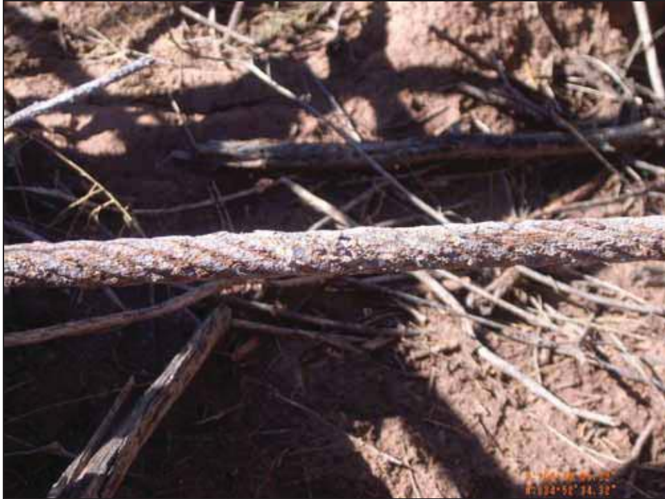
Figure 4.13. Steel cable connecting wooden pilings to one another.
