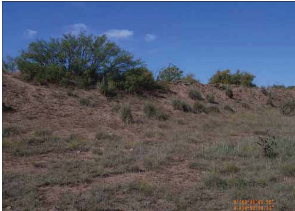
Figure 4.2. Earthen berm extending northwest from diversion, facing west.
