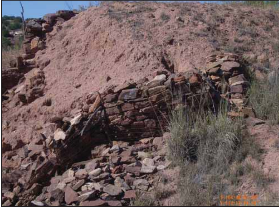
Figure 4.6. Eastern retaining walls at southern end of earthen berm, facing west.
