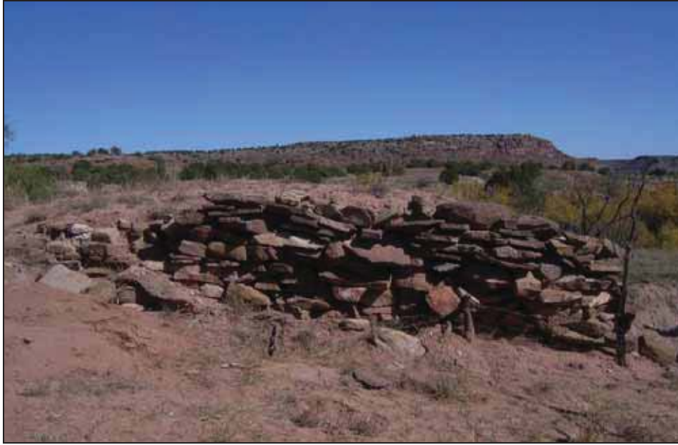
Figure 4.4. Western retaining wall, facing east.
