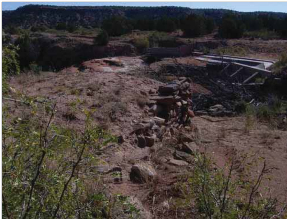
Figure 4.5. Western retaining wall, facing southeast.
