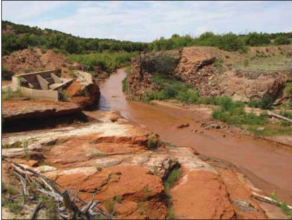
Figure 2.1. Overview of the diversion structure, looking west.
