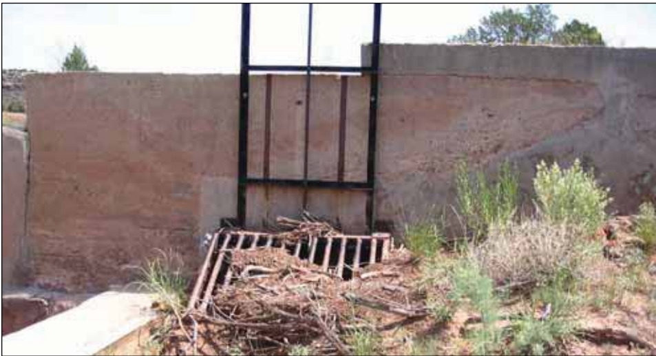
Figure 4.35. View of headgate, facing east.
