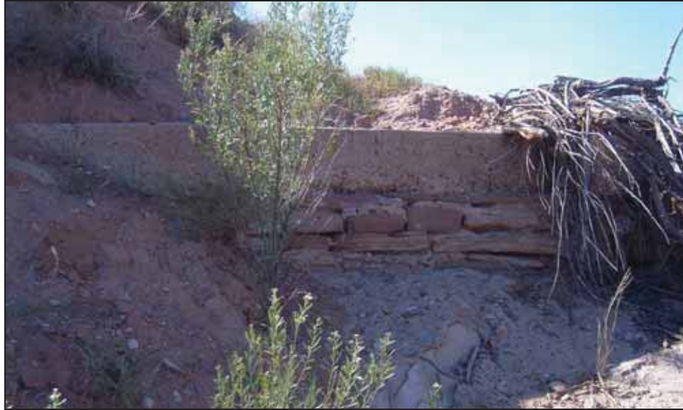
Figure 4.32. Segment of masonry diversion wall adjacent to northwestern corner of spillway.
