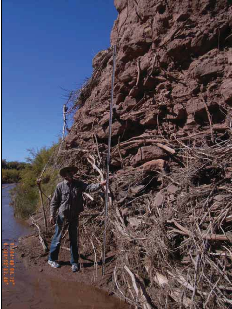
Figure 4.44. View of the northern cross-section of the diversion, showing base brush-dominated layer and multiple overlying layers of rock and brush.
