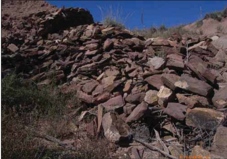
Figure 4.9. Remnants of masonry armor river bank, facing northwest (uphill) toward earthen berm.
