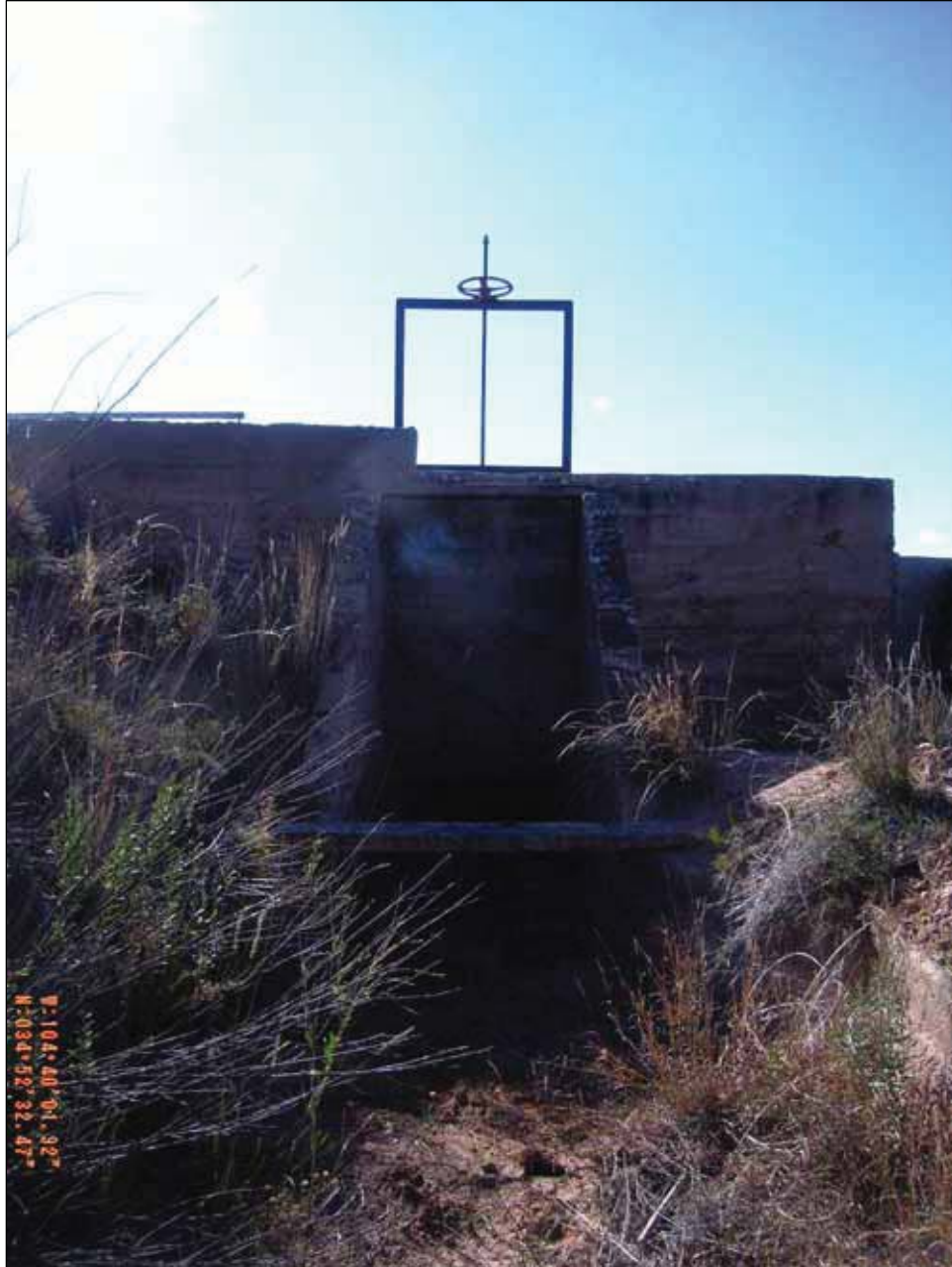
Figure 4.38. Headgate, facing east.
