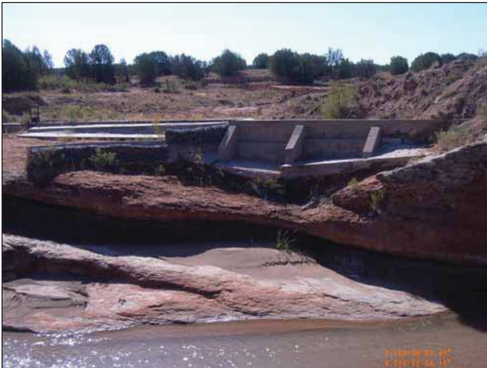
Figure 4.20. Overview of wall and gabion portions of spillway complex, facing south.
