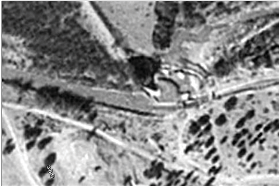
Figure 4.57. Aerial imagery of diversion complex dated May, 1997, showing location and shape of waterway leading to spillway and headgate. Imagery produced by U.S. Geological Survey and retrieved from Google Earth Pro (copyright 2009 Google and Europa Technologies).
