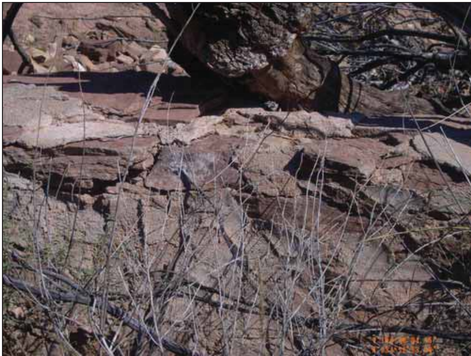
Figure 4.49. Close-up of masonry wall, showing concrete plastering, facing east.
