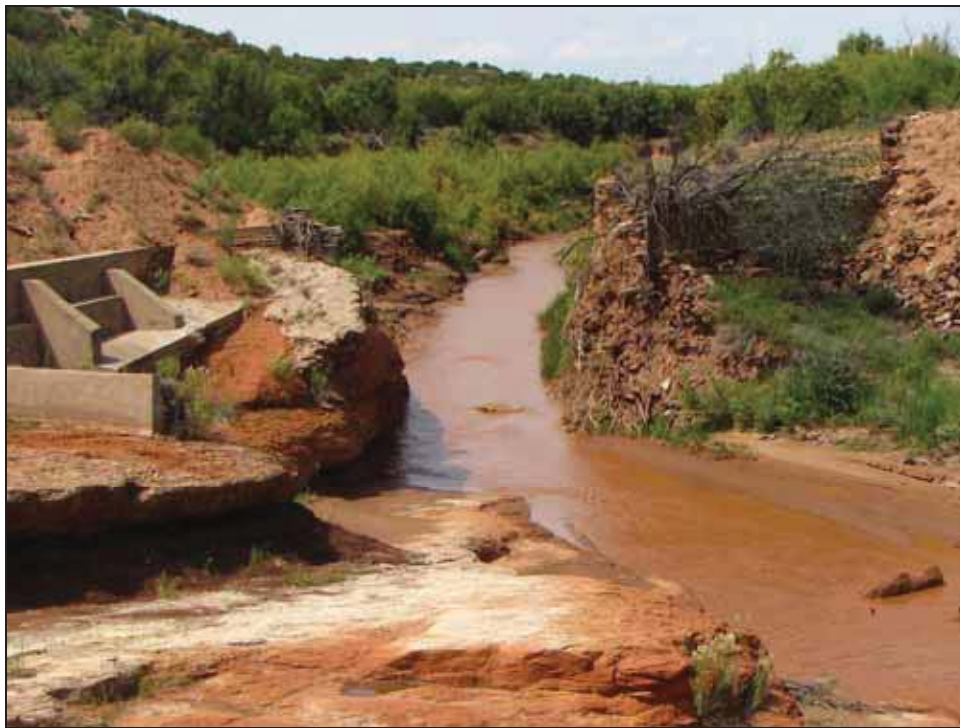
Figure 4.42. Overview of diversion complex, facing west.
