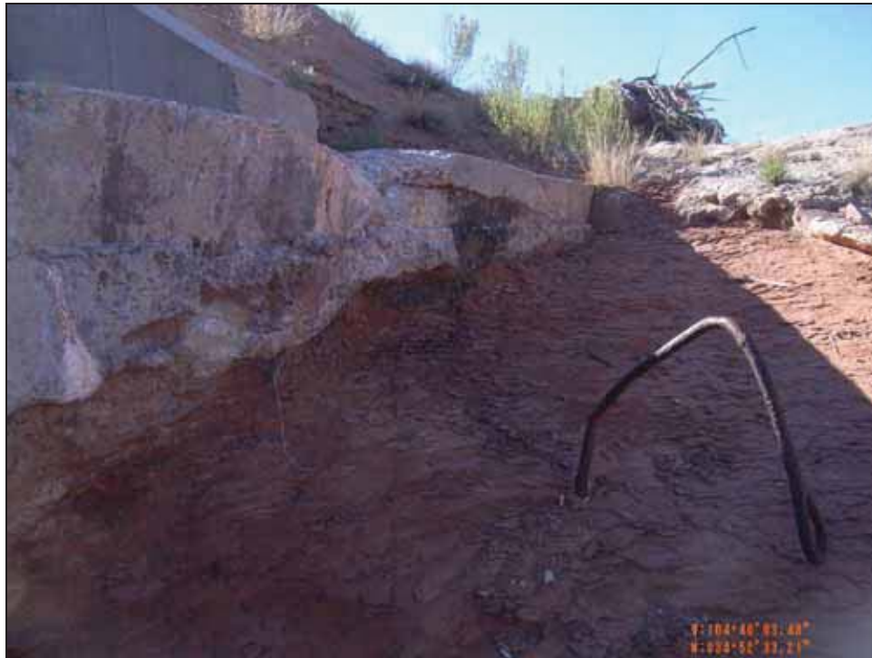
Figure 4.30. Metal rebar loop driven into bedrock adjacent to spillway structure.
