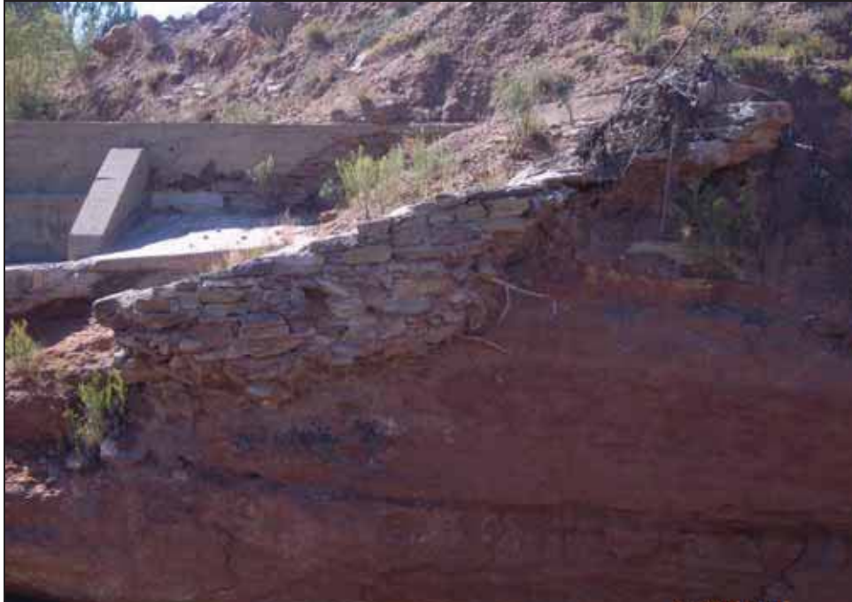
Figure 4.54. Remnants of masonry diversion wall and concrete-capped sandstone as viewed from the north side of the river, facing south.
