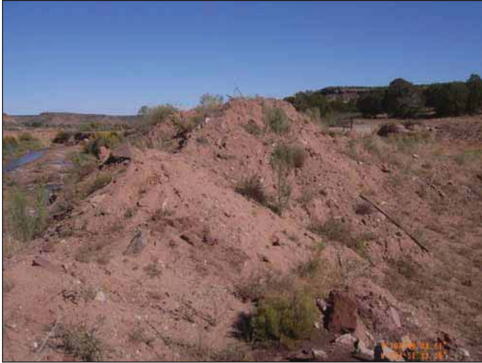
Figure 4.23. Large pile of rocks and dirt recently bulldozed over part of the spillway. This was done after the diversion was breached in 2006.
