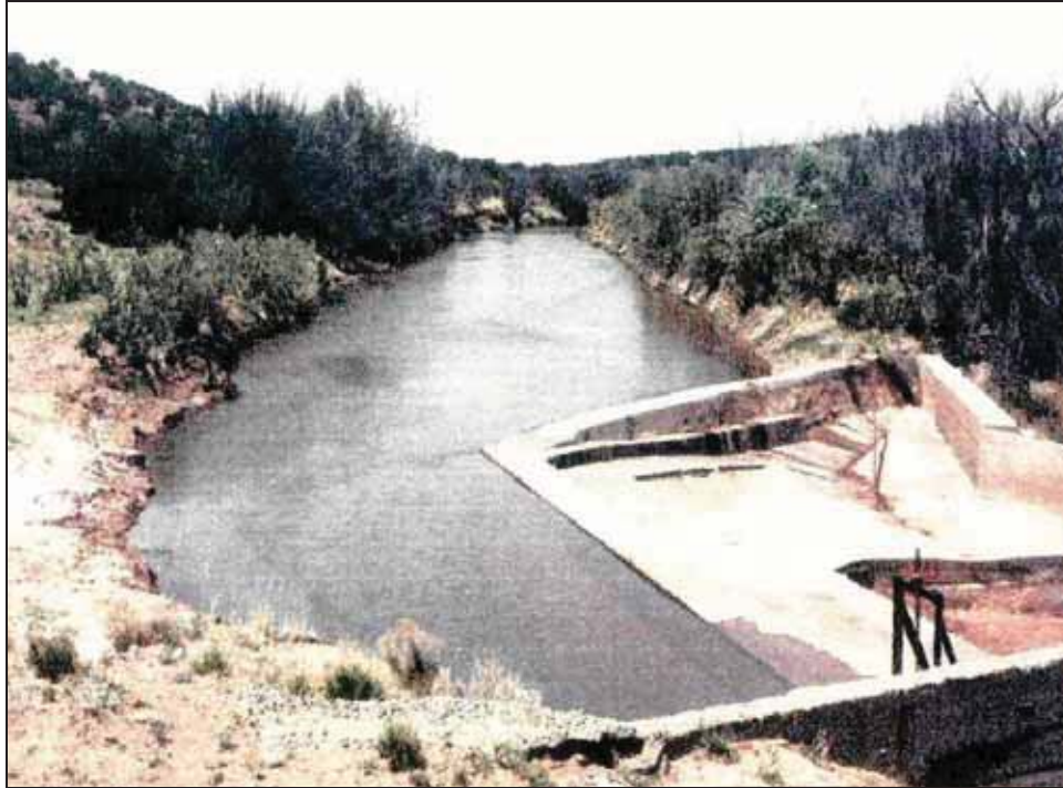
Figure 4.21. Diverted water approaching spillway and headgate, before the breach. (Photograph courtesy of the West Puerto de Luna Acequia Association).
