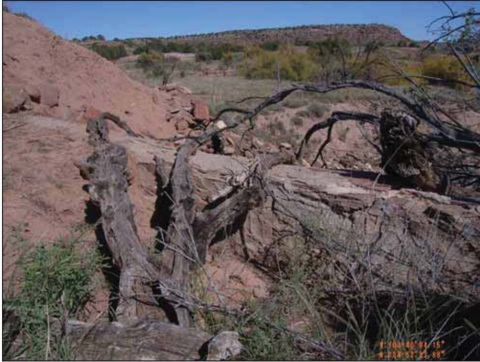
Figure 4.48. Northern segment of masonry diversion wall that once traversed the channel, facing east.
