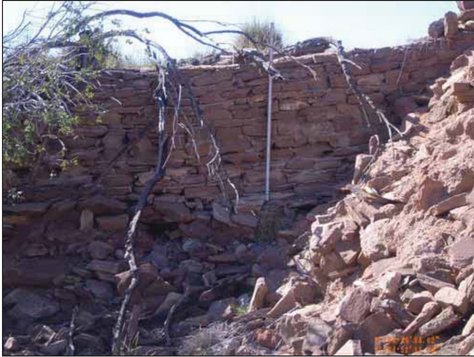
Figure 4.50. Northern segment of masonry diversion wall, facing west.
