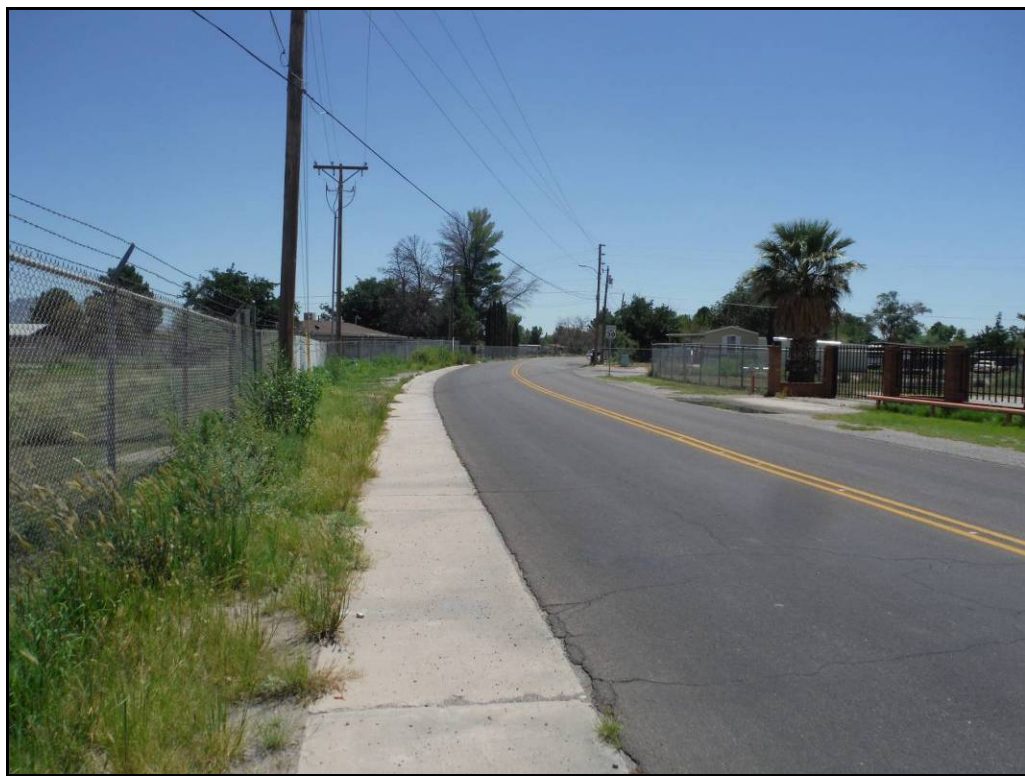
Figure 2. End of Phase II, EPWU-Canutillo Station, facing south.
