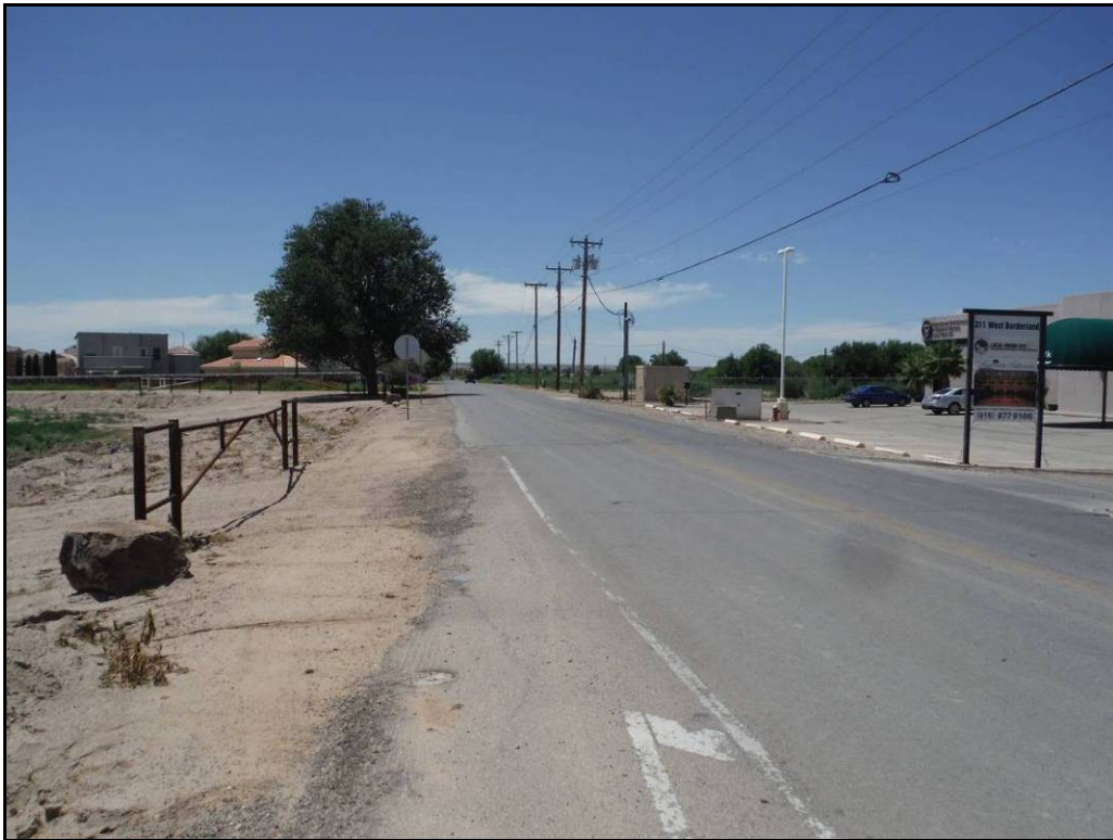
Figure 1. Beginning of Phase I on Rio Grande Bridge and East Borderland Road, facing west.
