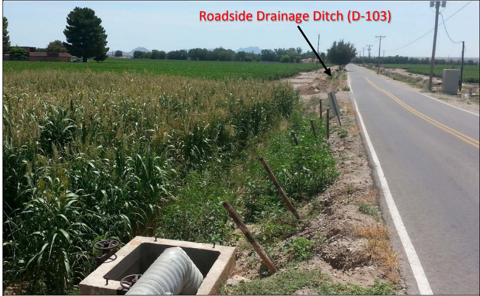
Phase I survey area along Strahan Road and south of irrigation canal. Photo Direction: south. Photo taken 8/18/2015.
