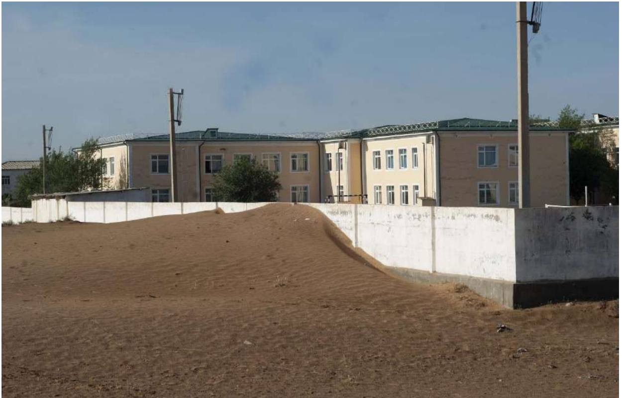
Fig.2.1.3. Results of sand encroachment, 2017 May
