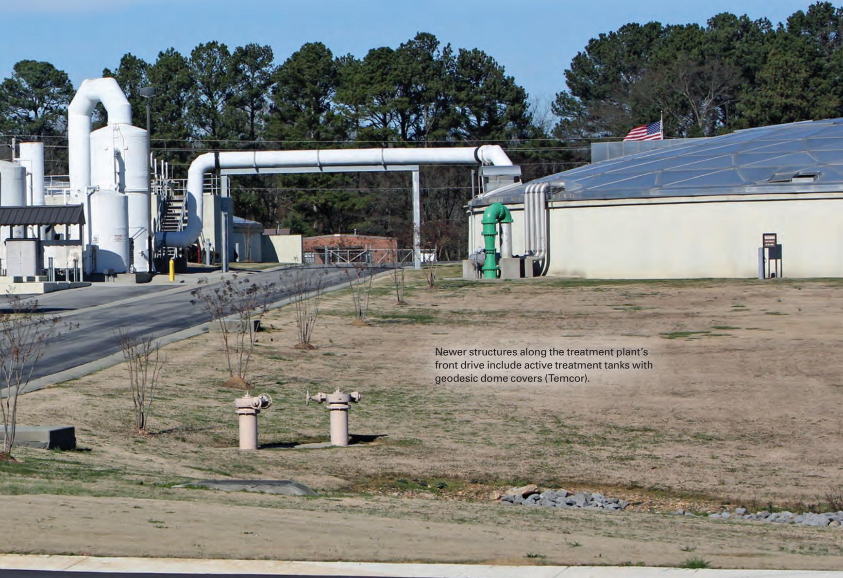
Newer structures along the treatment plant's front drive include active treatment tanks with geodesic dome covers (Temcor).
