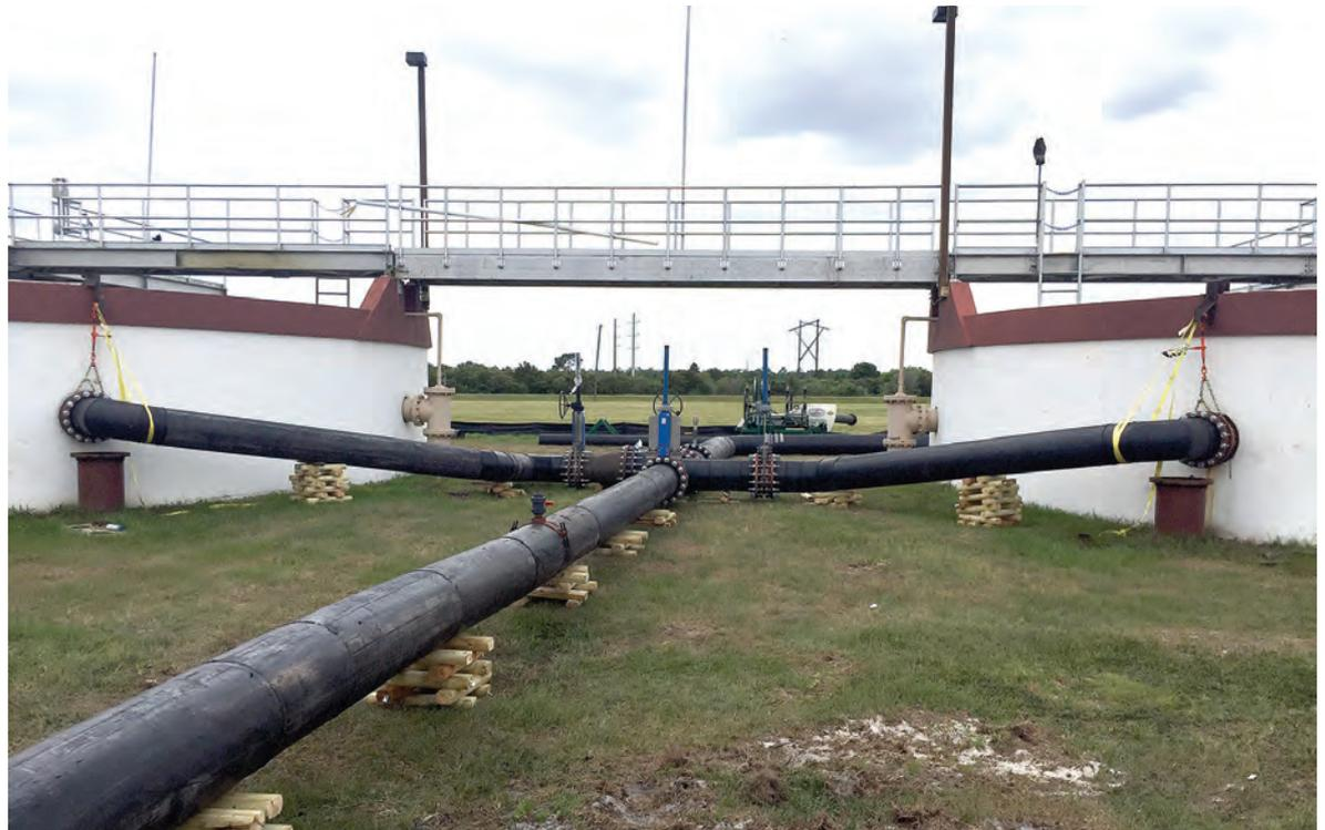
Flow from the aeration basins transfers by way of a 24-inch pipe to 18-inch lines that discharge to the east and west clarifiers at the back of the plant. In the background is the 18-inch crossover pipe that is used to help equalize the clarifiers during elevated flows.
