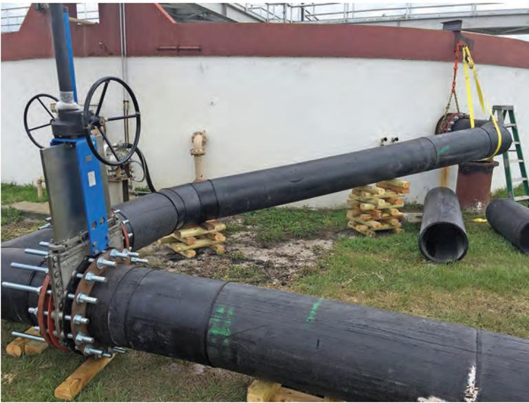
An 18-inch knife gate valve controls the flow from the 24-inch pipe feeding an 18-inch line to a clarifier.
