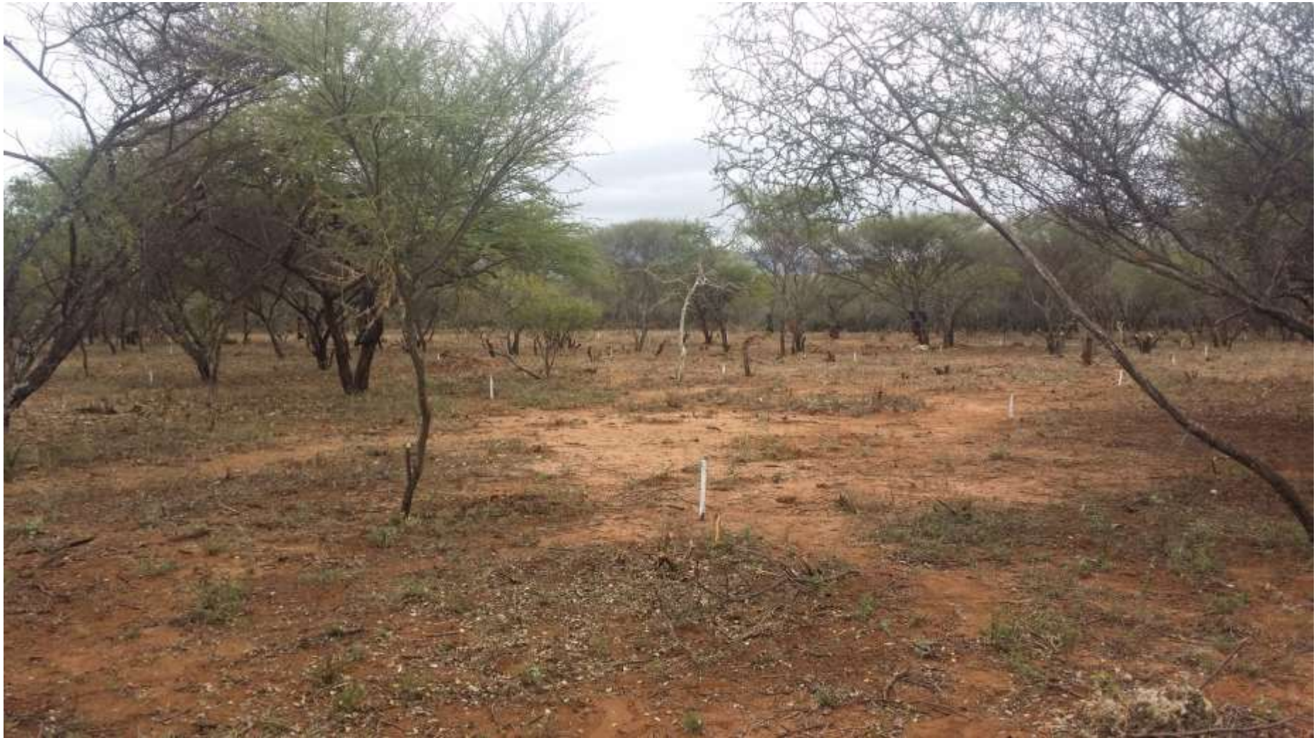
Operation 6.1: Scattered trees in the rangeland after thinning, undergrowth removed and surface cleared for grass growth
