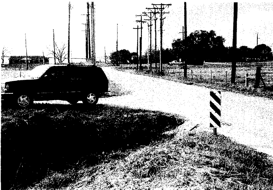
PHOTO 28 - LYTLE CANAL AT OLD FRIO ROAD
