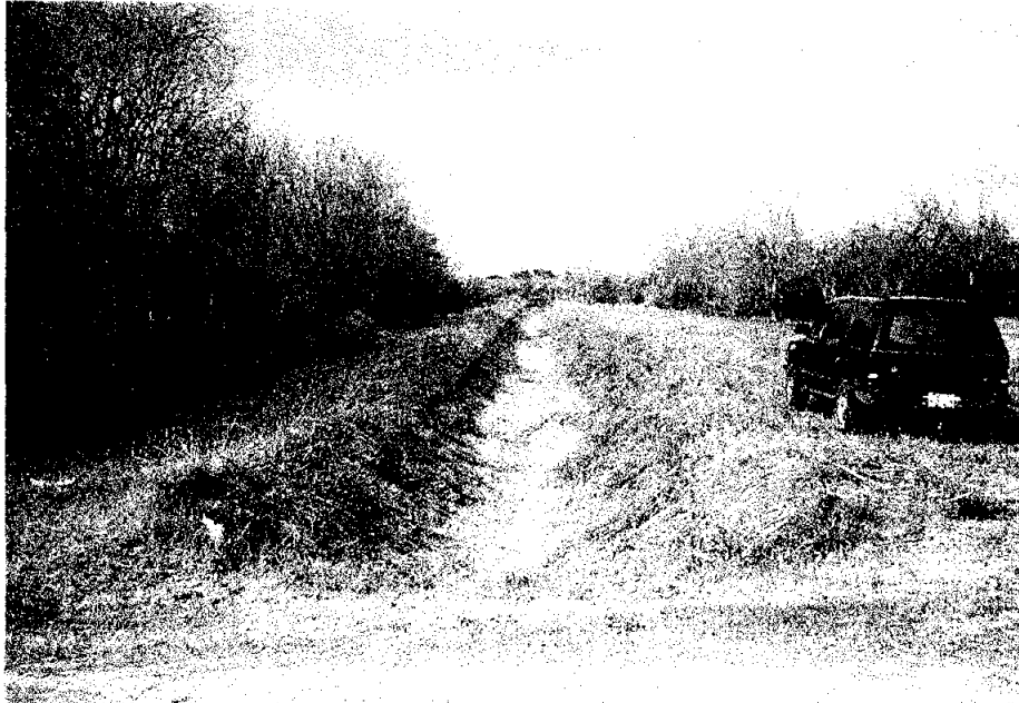
PHOTO 3 - TYPE C CANAL (D -2 Near E. Calame Rd.)
