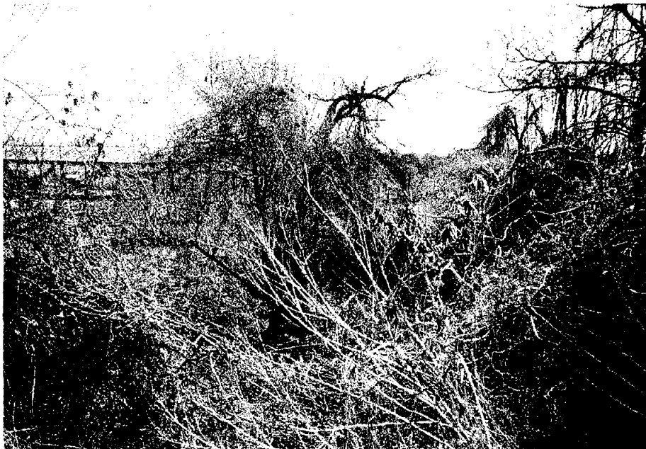
PHOTO 16 - OVERGROWN CANAL (D-2 at Dubose Lake)
