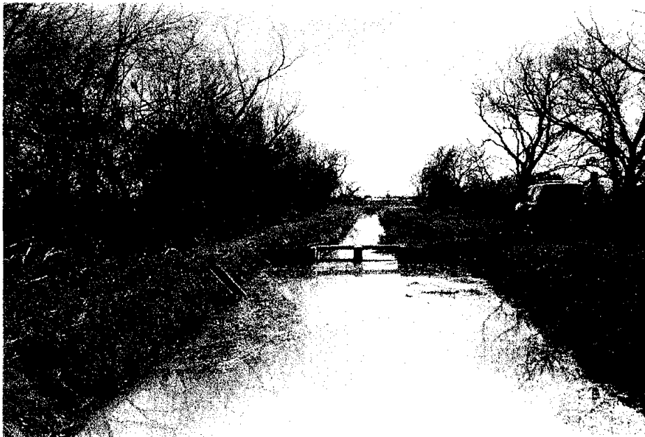
PHOTO 4 - TYPE D CANAL (Beyond Check, Natalia Canal)
