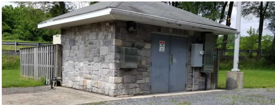
Figure 3-3: Exterior of Existing Scott Road Pump Station Building Structure
