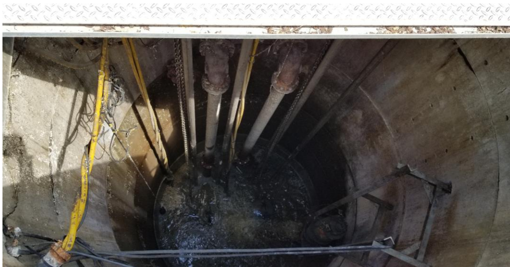
Figure 3-2: Interior of the Existing 8 foot Diameter Wet Well
