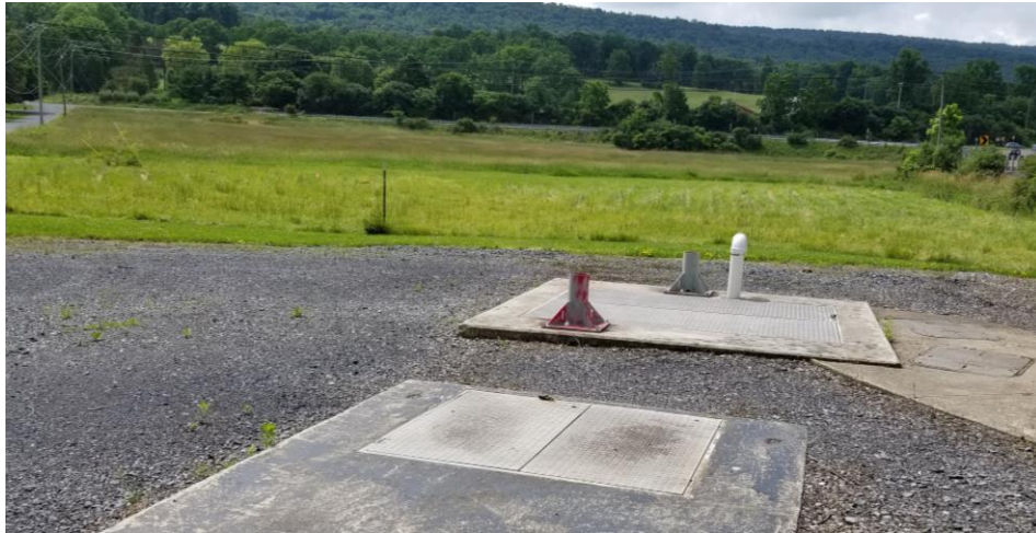
Figure 3-1: Existing Wet Well and Valve Vault at the Scott Road Pump Station
