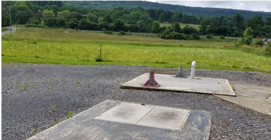
Figure 3-1: Existing Wet Well and Valve Vault at the Scott Road Pump Station
