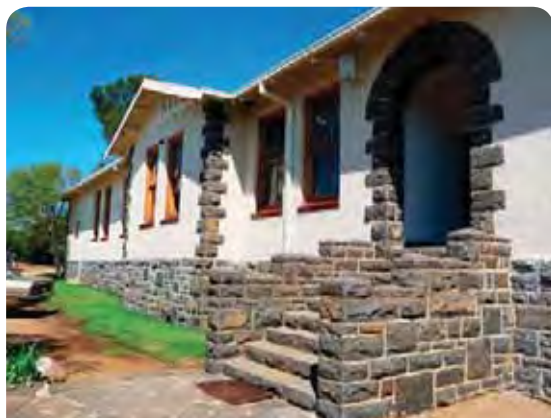
Renovated main building of the Boyden Observatory.
