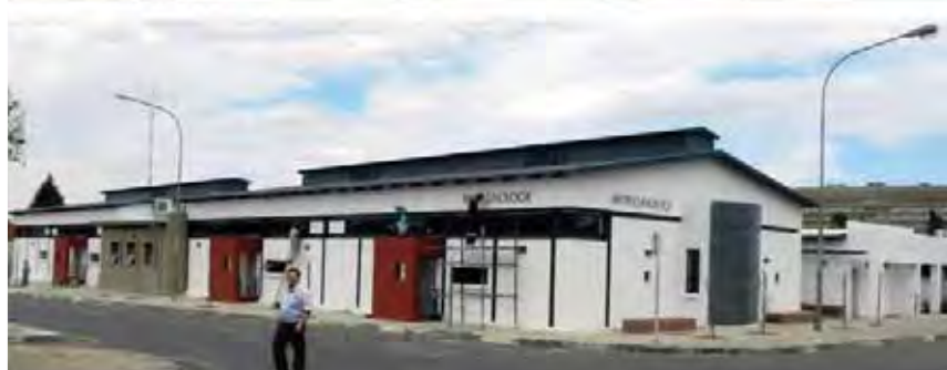
The new undergraduate laboratories: before start of construction (top) and at completion (bottom).
